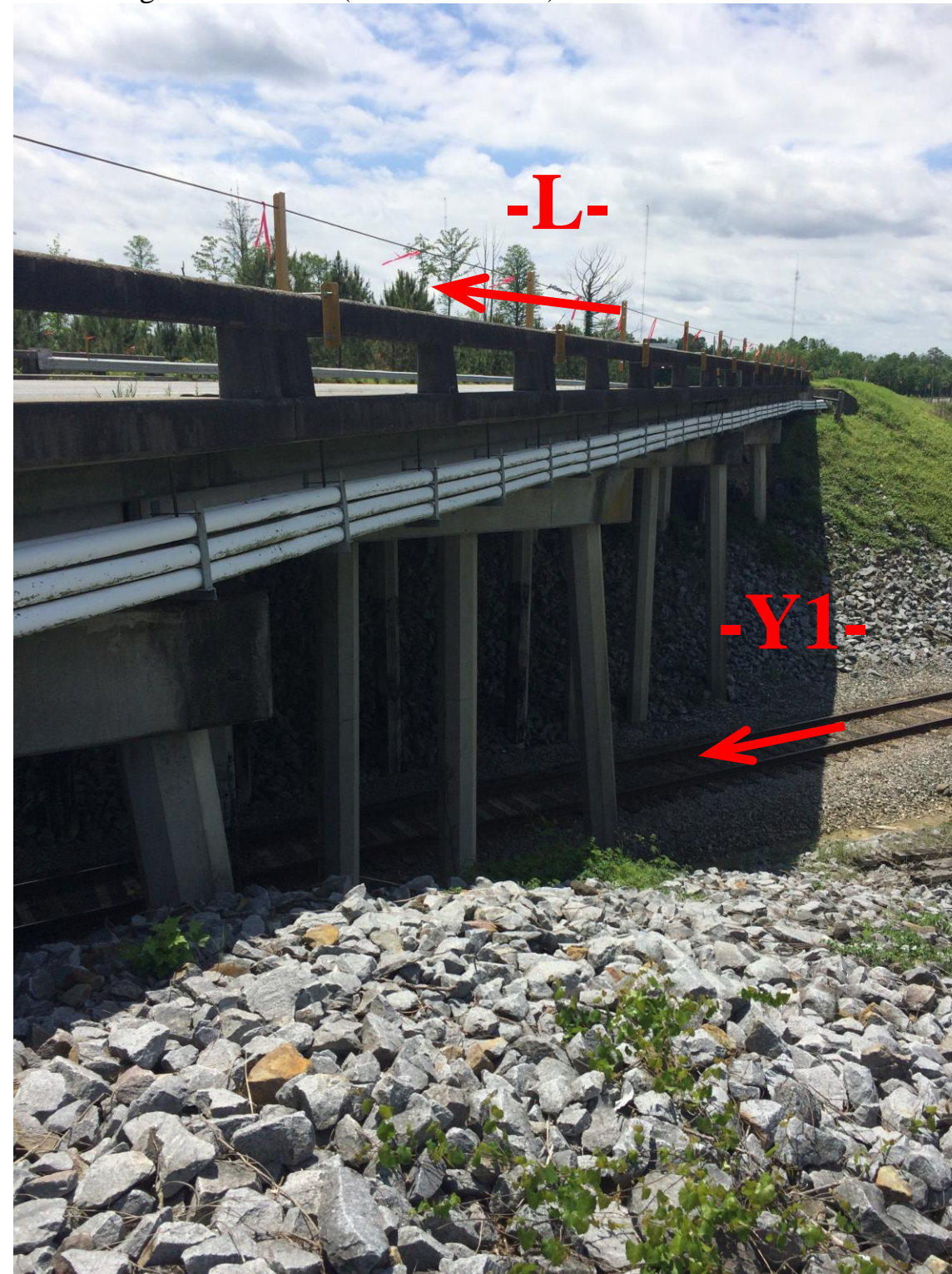
Bridge No. 3 on -L- (US 17 Business) over Norfolk Southern RR
