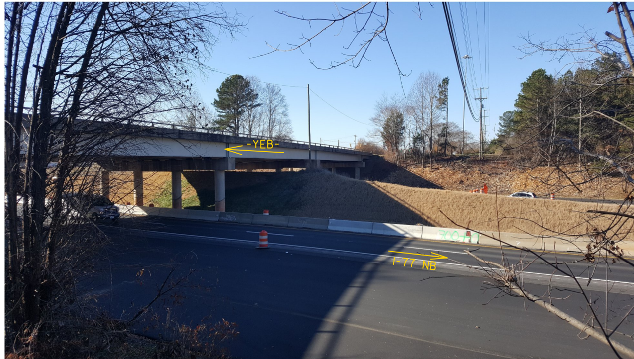
Photo No. 1: View at existing Bent 2 looking west (downstation) on -YEB- (SR 2136)
