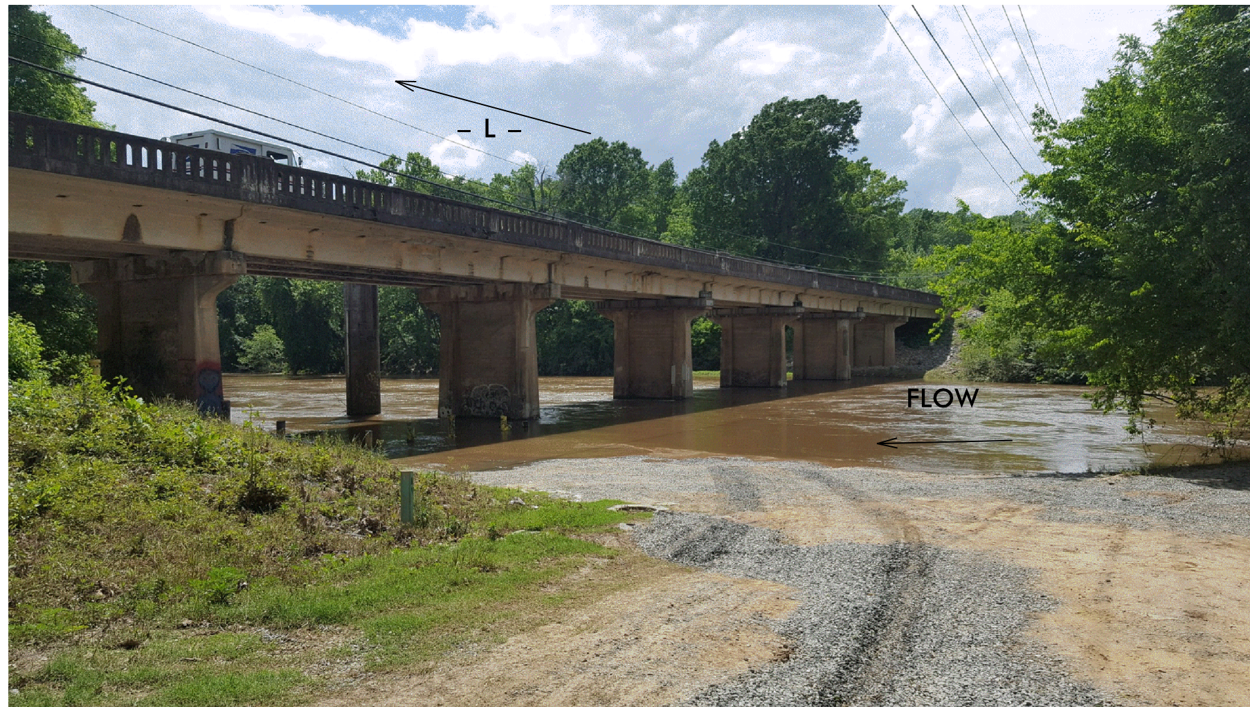
Looking west toward End Bent 1
