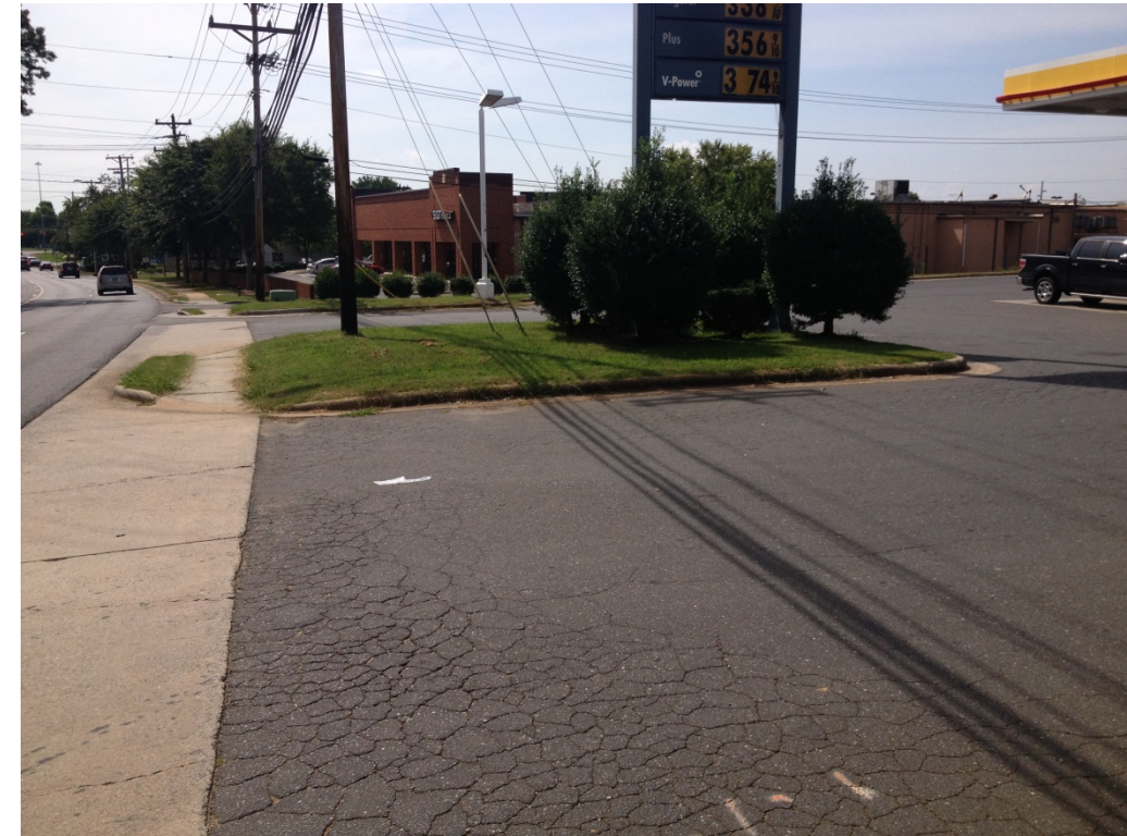
B. Photo of Shell site from east side of property, looking west.
