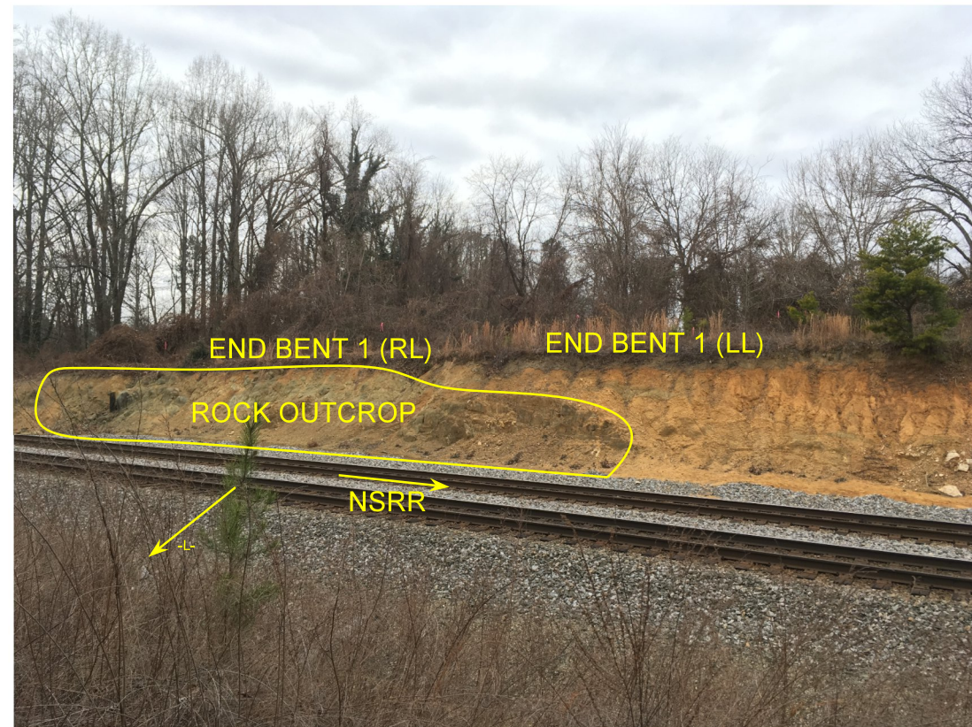
LOOKING DOWN STATION (WEST) FROM BENT 1 (LL) TO END BENT 1 (LL & RL)
