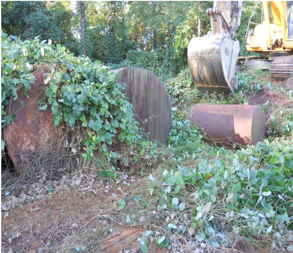
Photograph No. 10 View of clearing vegetation off of tanks.
