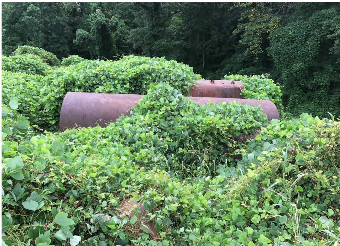
Photograph No. 5 View of tanks (former USTs) located on the south side of the site.
