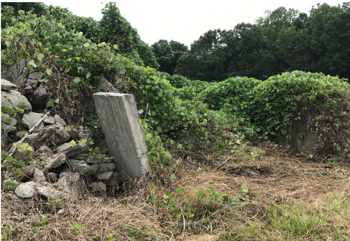
Photograph No. 3 View of typical piles of concrete, brick, and rock debris.
