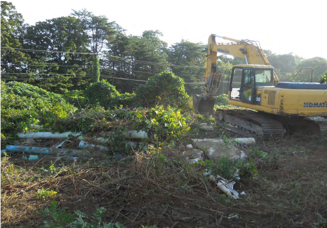
Photograph No. 7 Clearing and grubbing the site.
