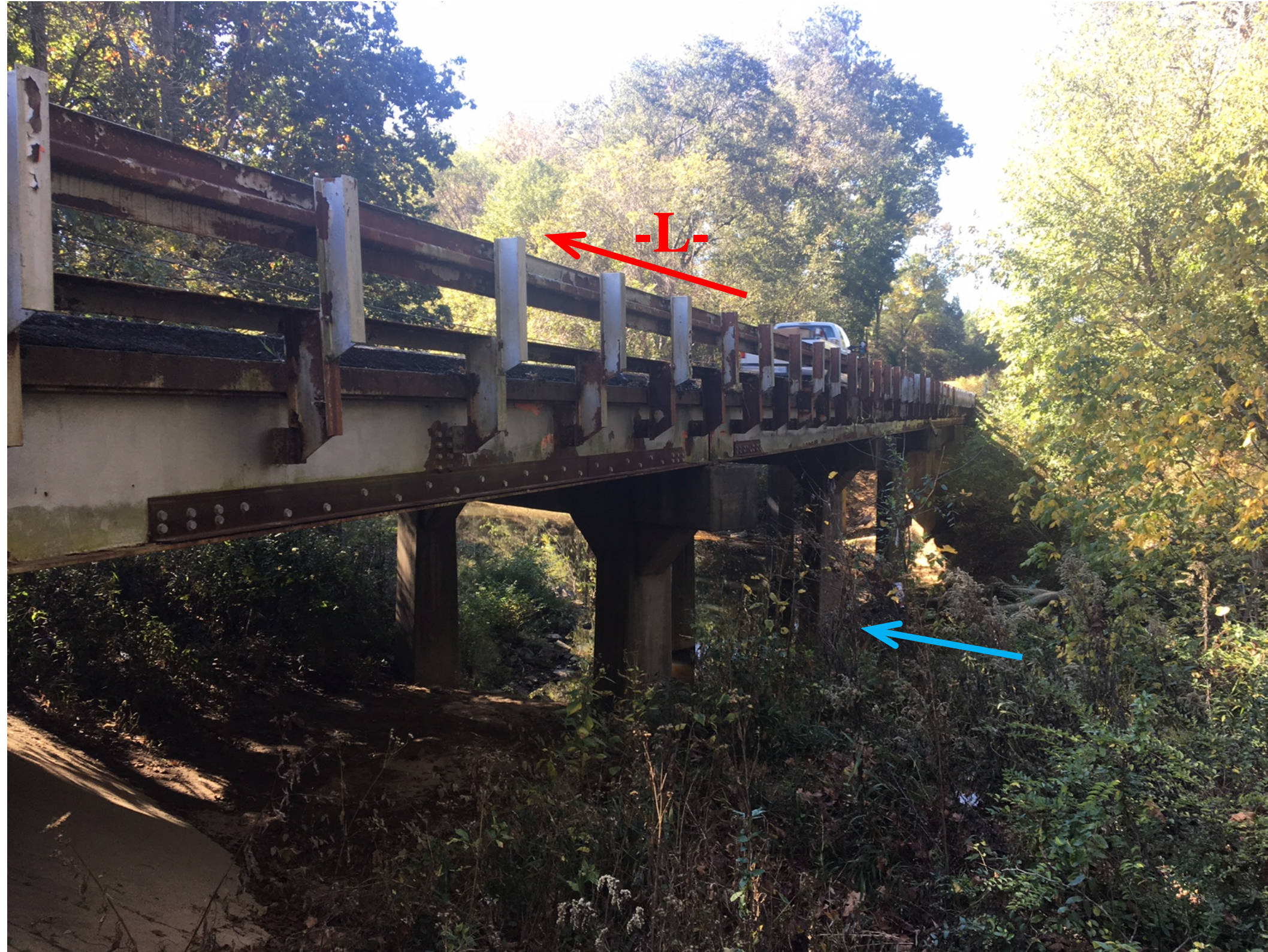
Looking Southwest towards End Bent 1
