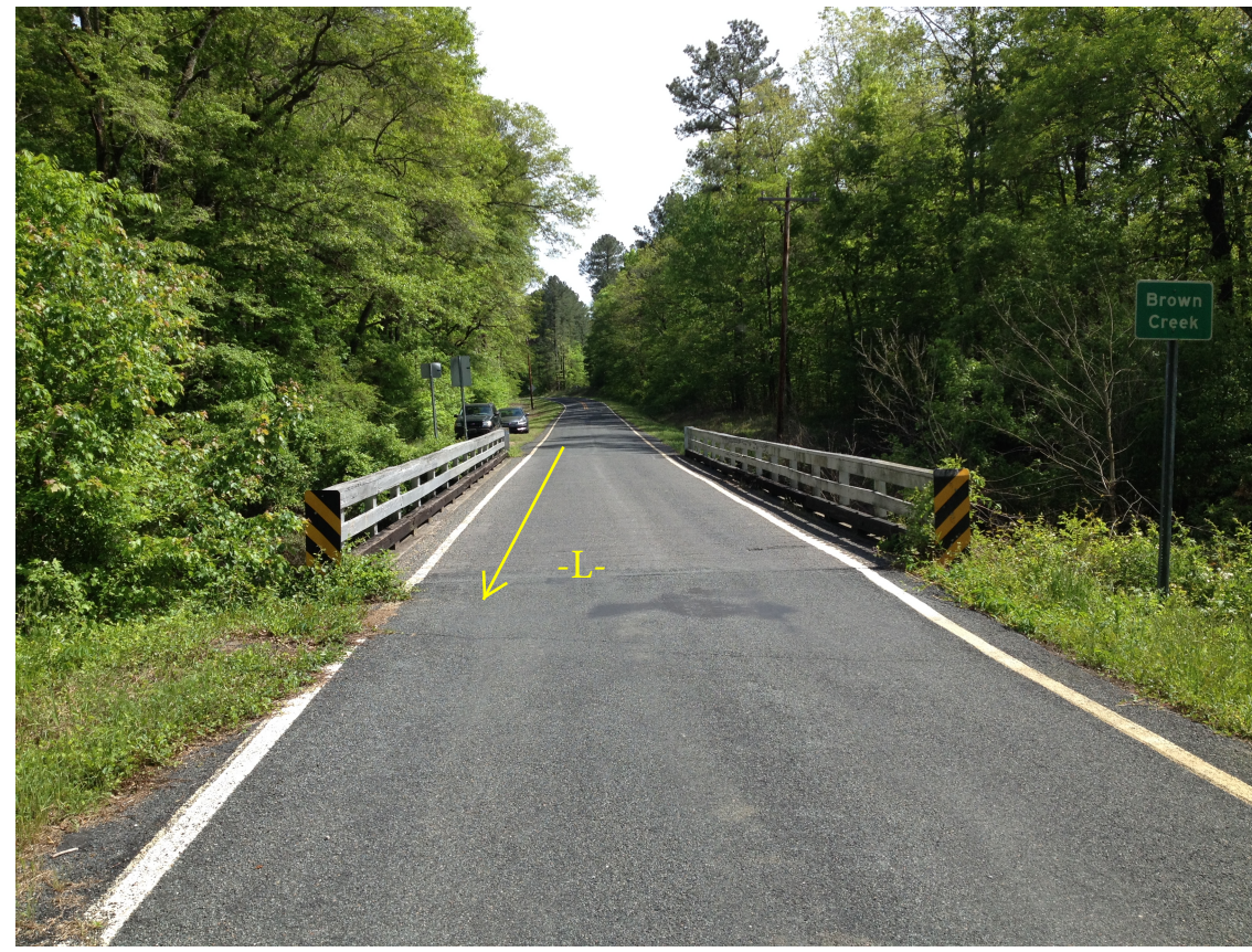
VIEW OF BRIDGE 008 LOOKING SOUTH
