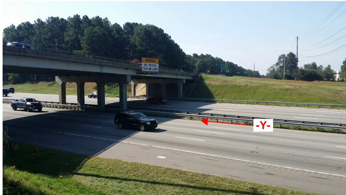
Photo 1: Looking Southeast towards End Bent 1 and Bent 1
