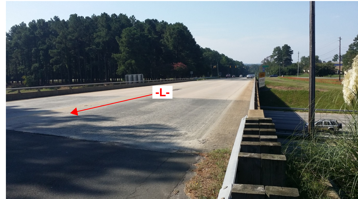
Photo 2: Looking South along SR1002
