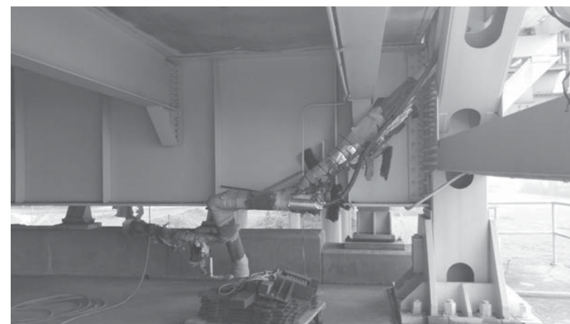
EXISTING CONDITIONS PHOTOGRAPH #6 NOT TO SCALE
