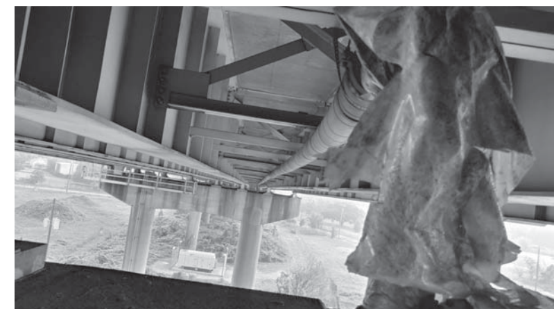
EXISTING CONDITIONS PHOTOGRAPH #7 NOT TO SCALE
