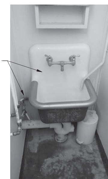
EXISTING CONDITIONS PHOTOGRAPH #1 NOT TO SCALE
