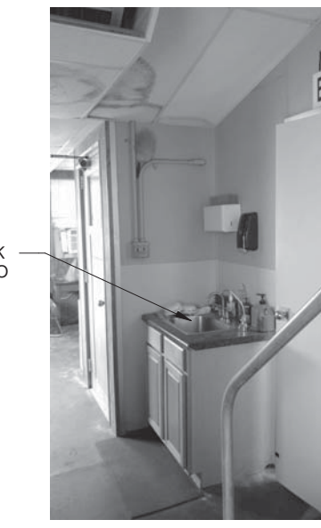
EXISTING CONDITIONS PHOTOGRAPH #5 NOT TO SCALE
