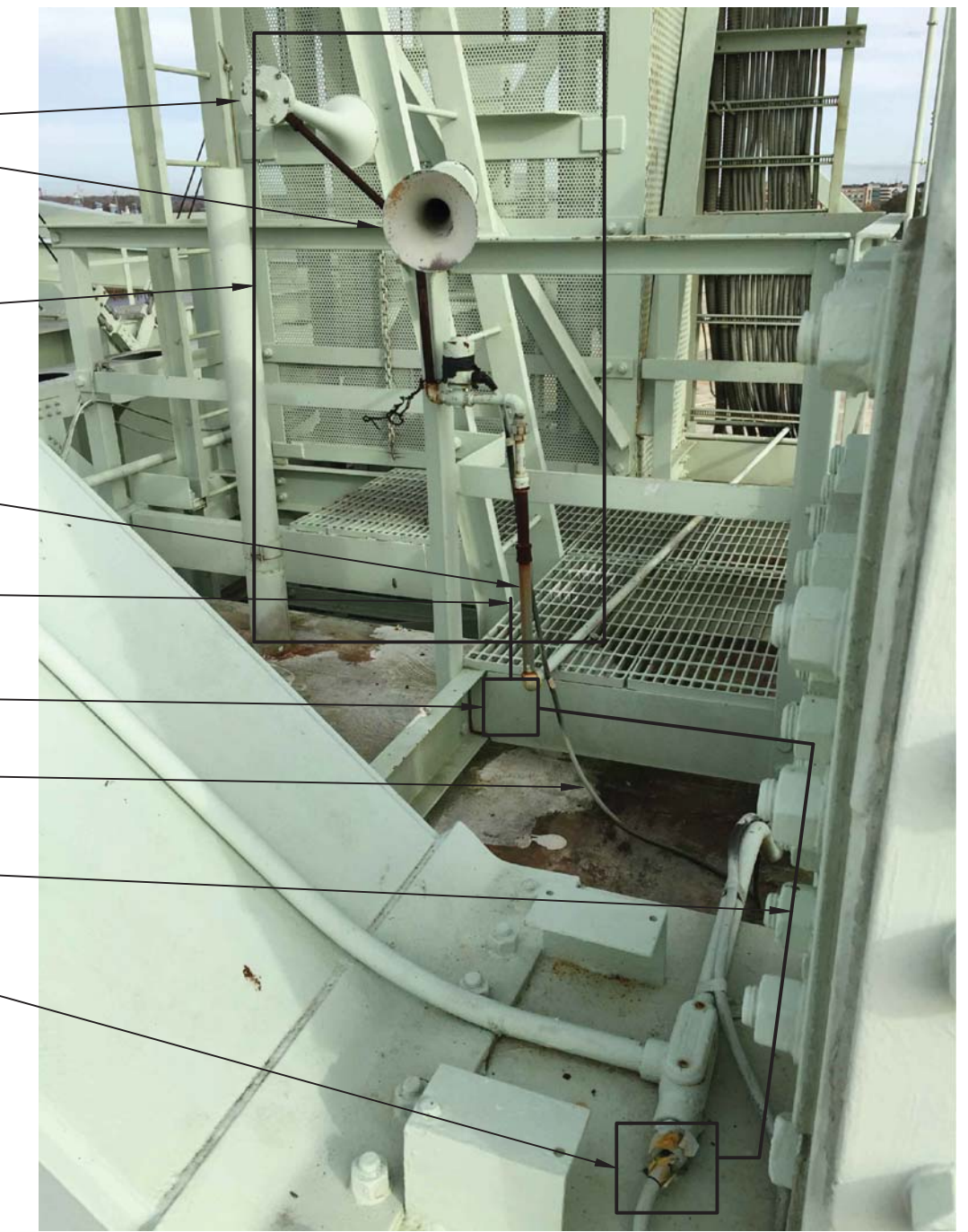
AIR HORN REPLACEMENT DETAIL NO SCALE
