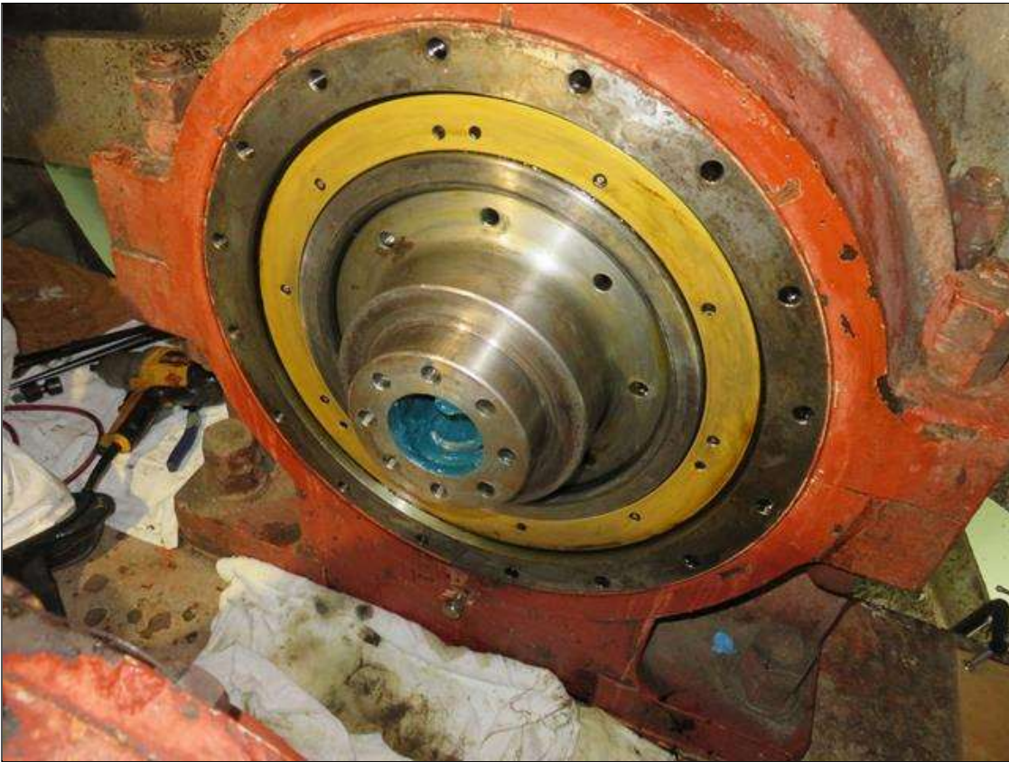
SOUTH EAST ROOM SOUTH SIDE INNER TRUNNION FACE DISASSEMBLED.
