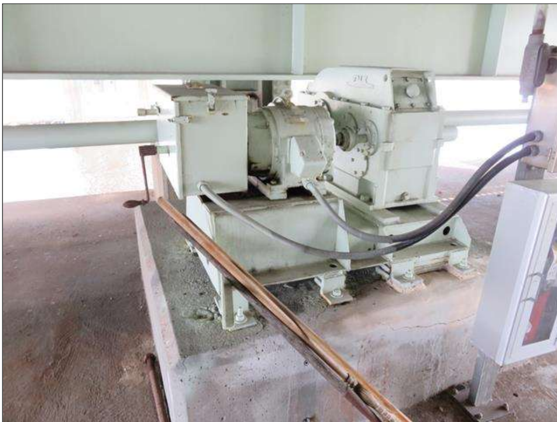
WEST LOCK DRIVE
