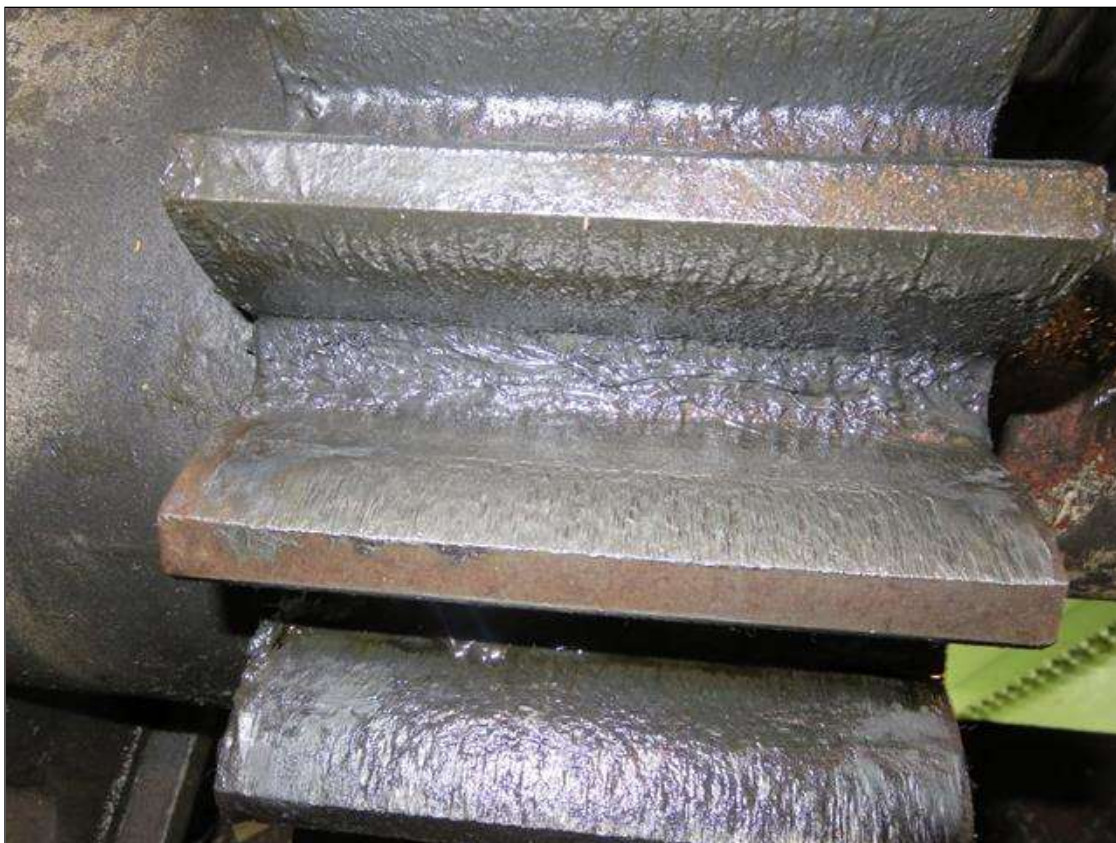
GEAR 276 HAS 1/32" GROOVES IN OPEN AND CLOSING SIDE OF TOOTH SOUTH WEST ROOM (WEST TOWER)
