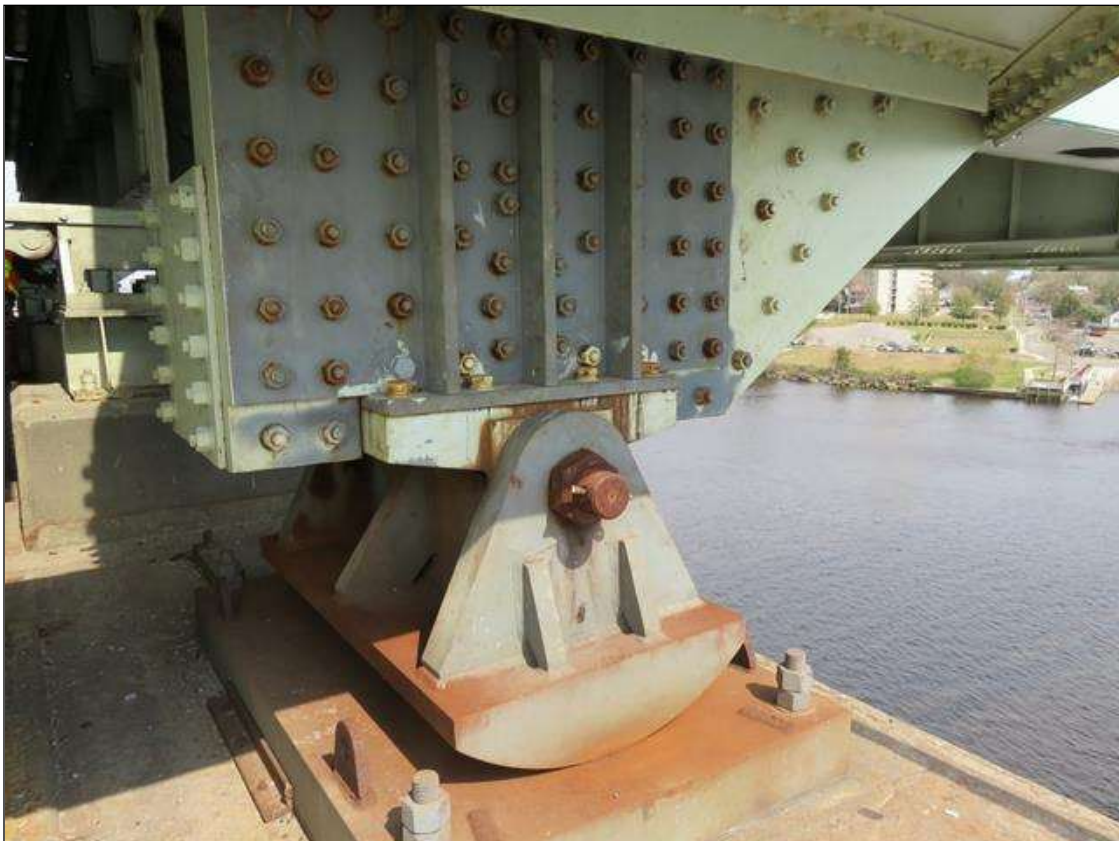
OUTSIDE FACE OF SOUTH WEST BEARING ASSEMBLY.
