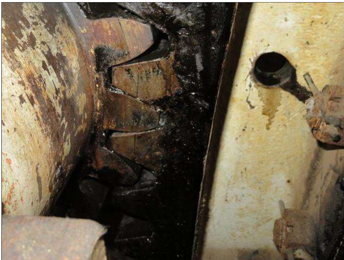
BACKLASH OF .072 WAS MEASURED FOR #277 & 271-1 GEARS IN SOUTH EAST ROOM.
