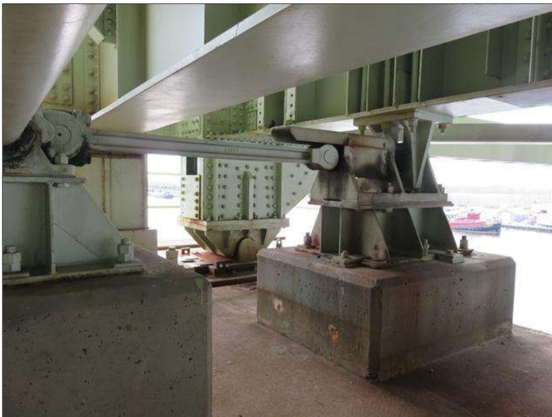
LOCK MACHINERY EAST TOWER.
