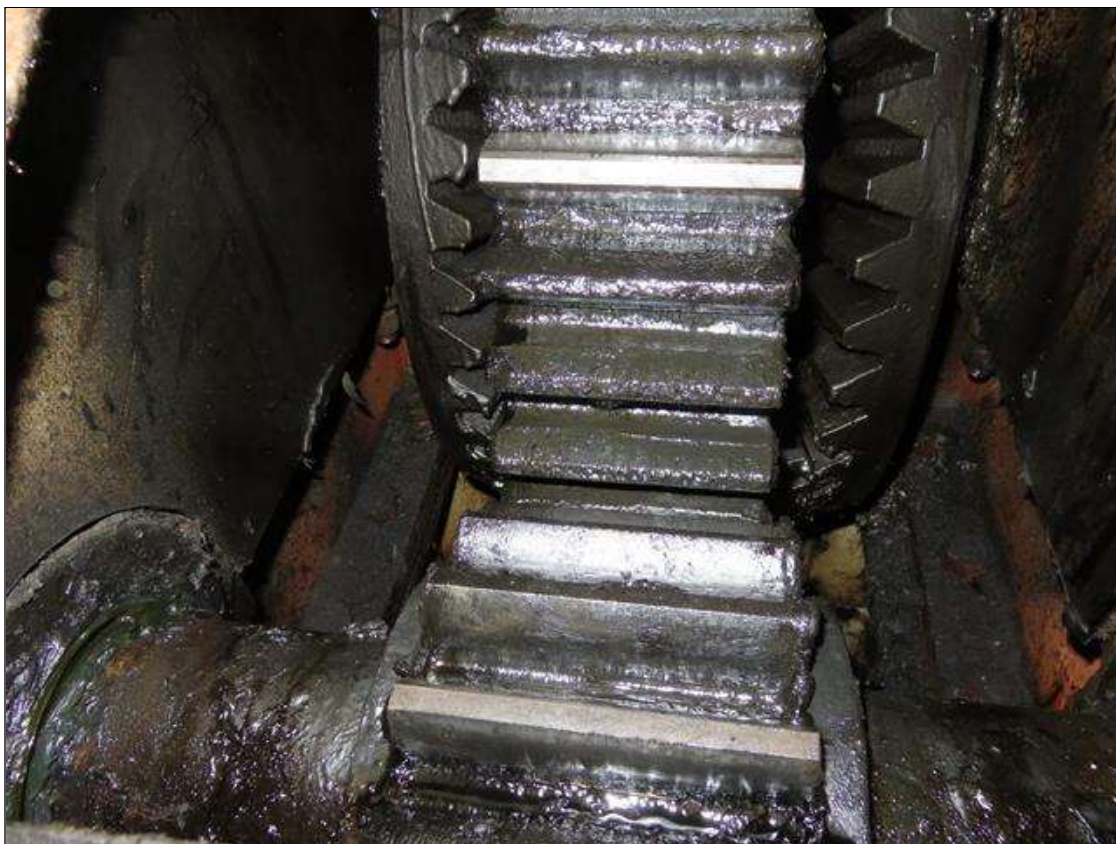
GEARS 357 & 278 SOUTH WEST ROOM (WEST TOWER)
