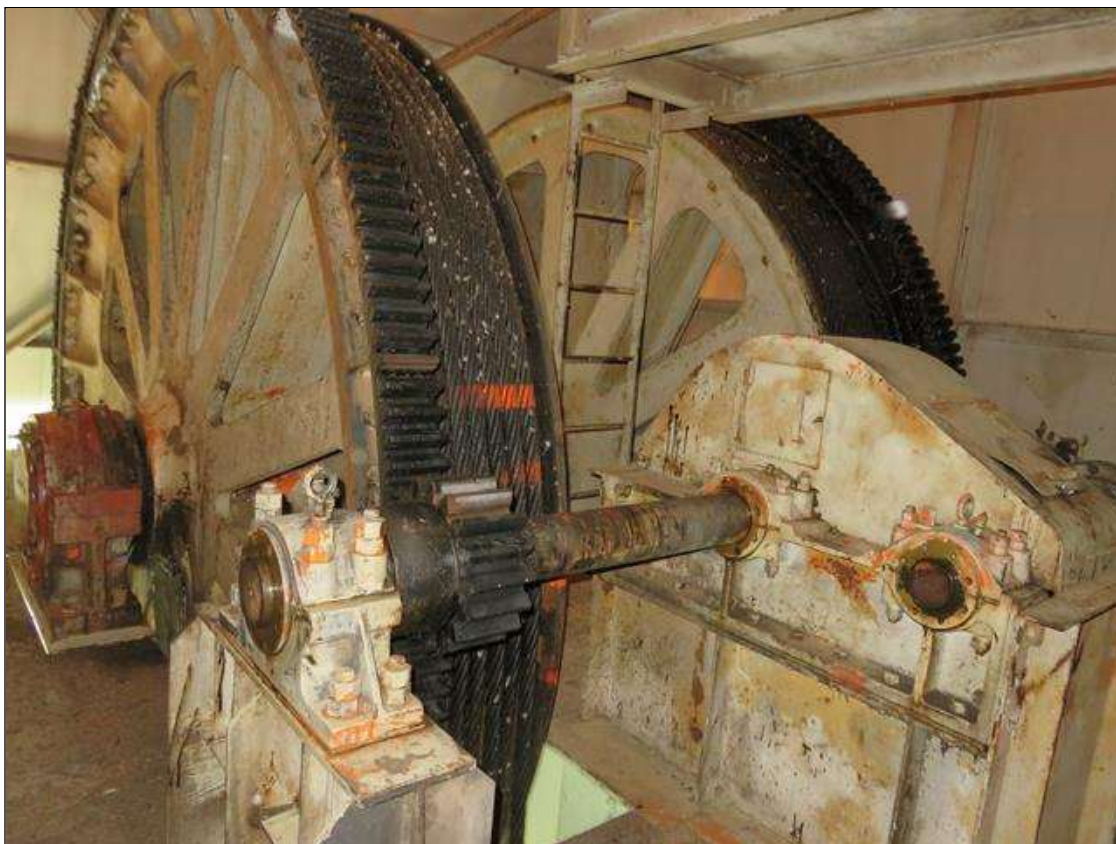
OPERATING MACHINERY IN SOUTH EAST ROOM.
