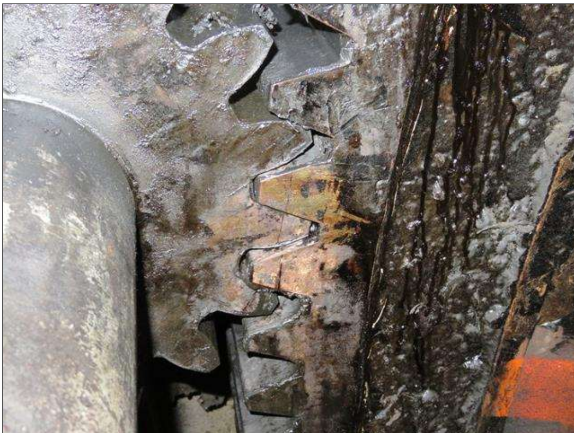
BACKLASH OF .084 WAS MEASURED FOR #276 & 271-2 GEARS IN SOUTH EAST ROOM.
