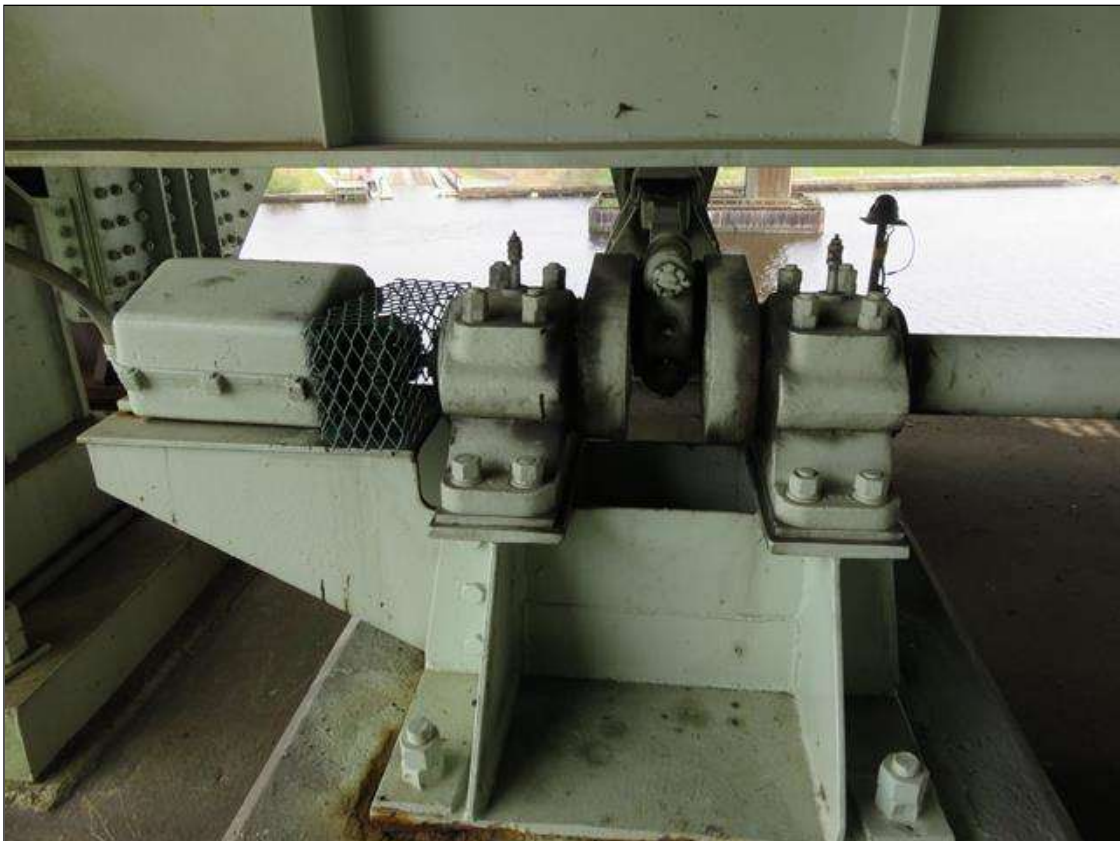
NORTH TOWER LOCK (DIFFERENT VIEW)
