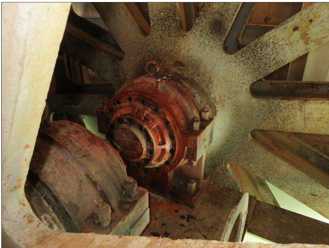
SOUTH EAST ROOM SOUTH INNER TRUNNION REASSEMBLED AFTER UT INSPECTION.
