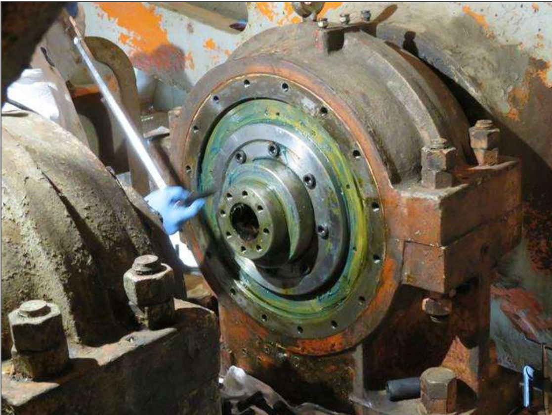
NORTH WEST ROOM INNER SOUTH TRUNNION BEING REASSEMBLED BY BRIDGE CREW.
