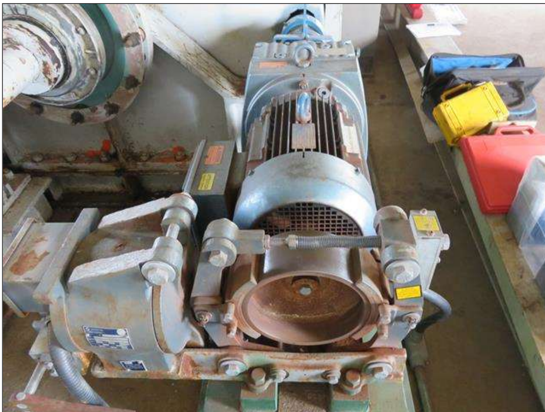
EAST AUXILARY DRIVE GEAR MOTOR BRAKE (GOOD)
