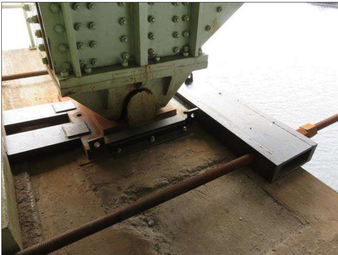
EAST TOWER FIXED SHOE WITH REINFORCED SUPPORT.
