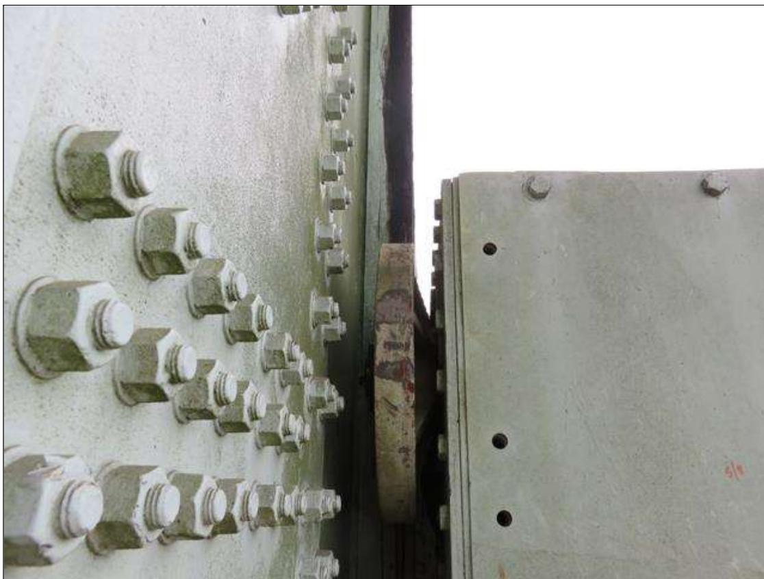
GUIDE WHEEL ON NORTH EAST SIDE FROZEN.
