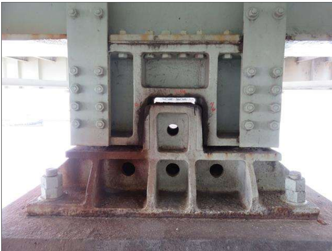
EAST SIDE TRANSVERSE CENTERING SHOE.
