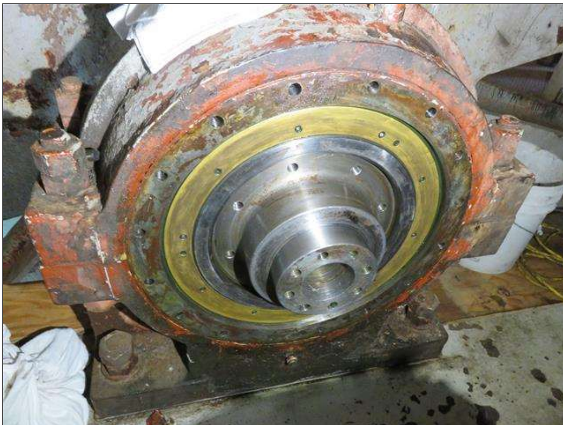
SOUTH WEST INNER TRUNNION DISASSEMBLED FOR ULTRA SONICS INSPECTION. (SOUTH SIDE)
