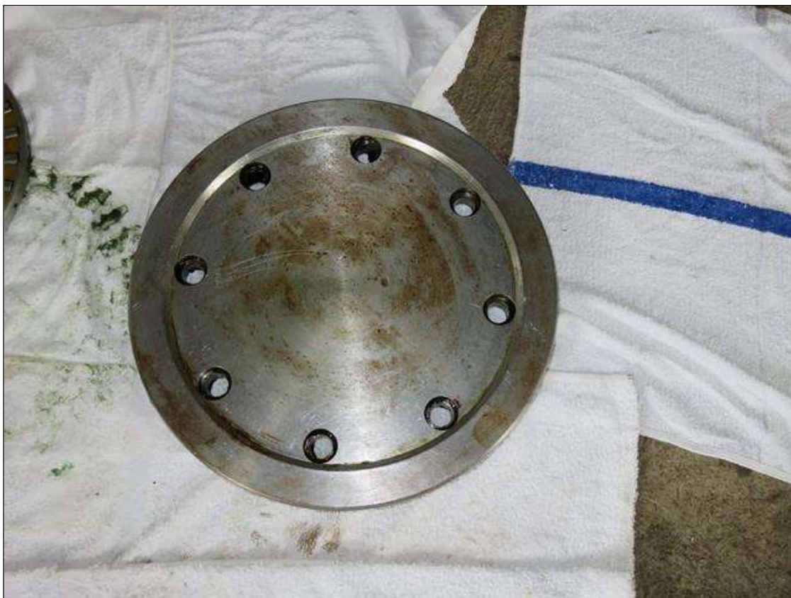
NORTH WEST ROOM OUTSIDE SOUTH TRUNNION INNER PLATE. (FAIR MINOR SURFACE STAINING/ SURFACE RUSTING WITH NO SECTION LOSS.)
