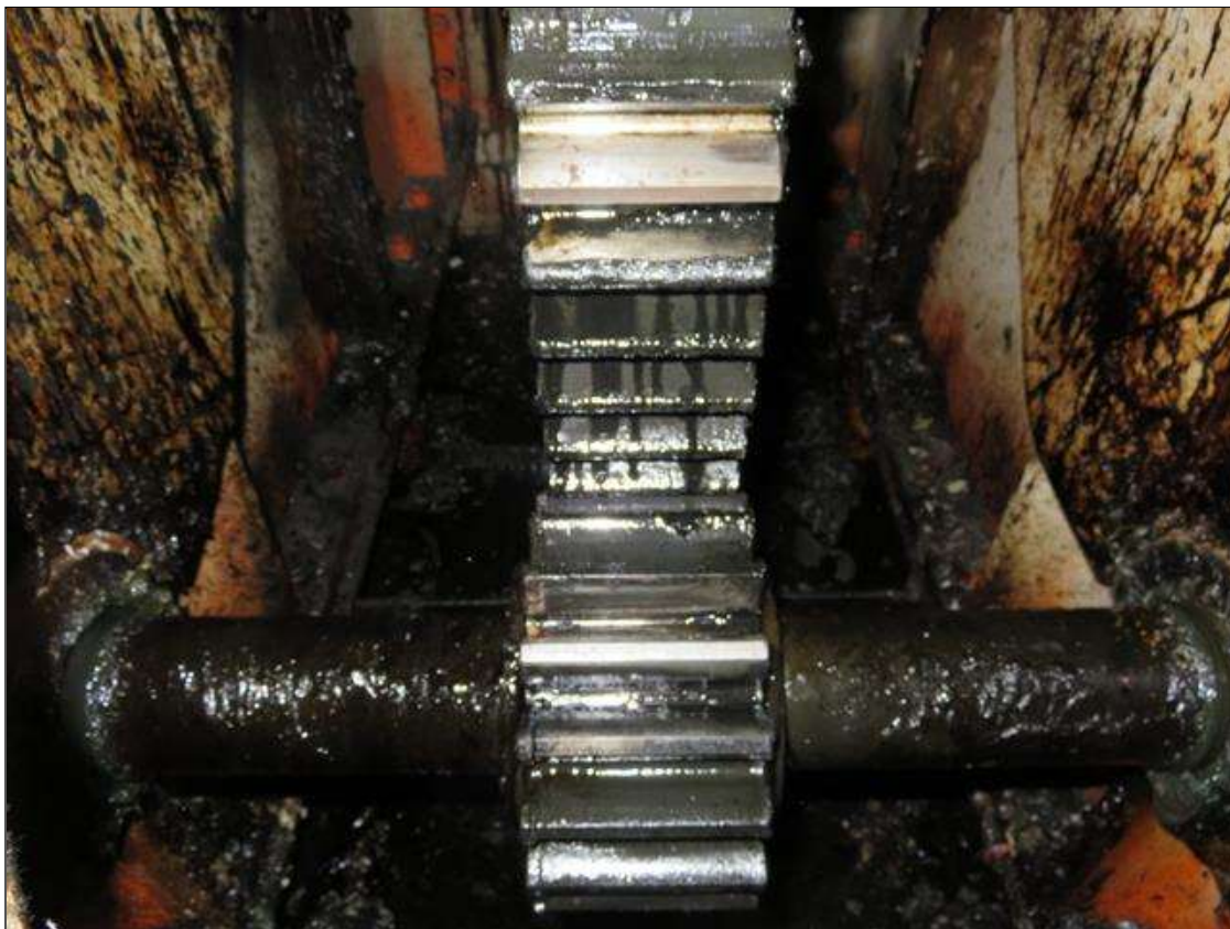
GEARS #279 & 358 OPERATING MACHINERY EAST TOWER (GOOD CONDITION)
