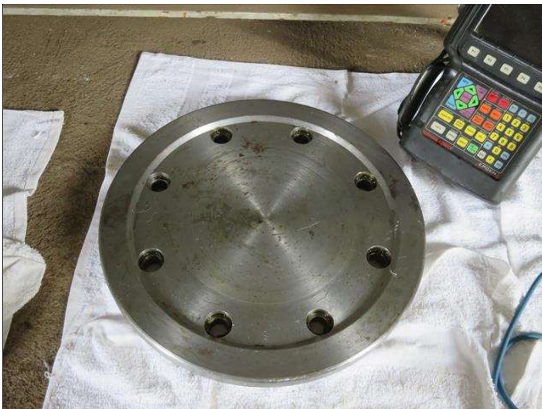
SOUTH WEST ROOM OUTSIDE SOUTH TRUNNION INNER PLATE. (GOOD NO PROBLEMS FOUND)
