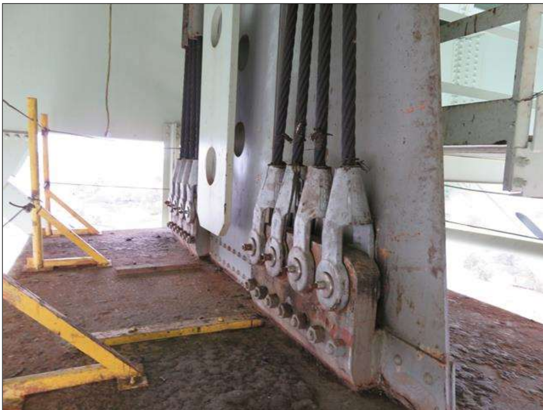
CABLE ATTACHMENT TO COUNTER WEIGHT (EAST TOWER)
