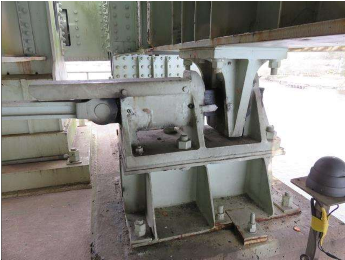
NORTH WEST TOWER & LOCK
