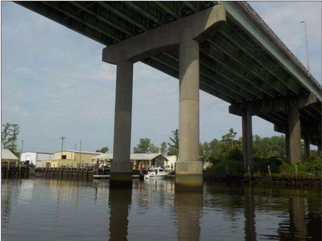
BENT 13, SPAN 14 SIDE
