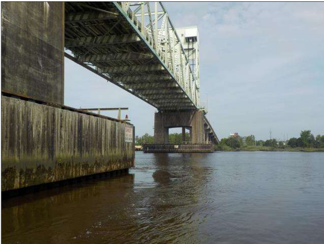
LOOKING WEST ALONG NORTH SIDE
