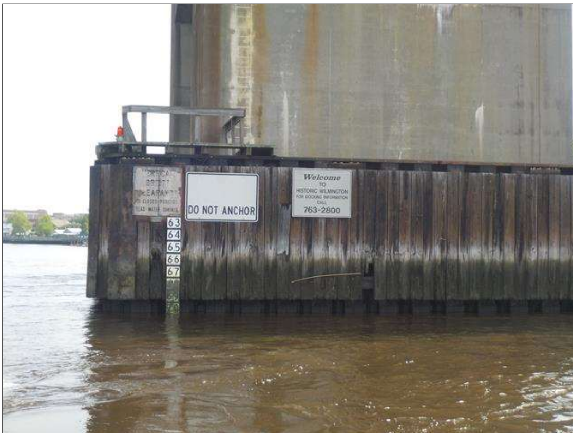
BENT 17, SIGNS, SOUTH SIDE
