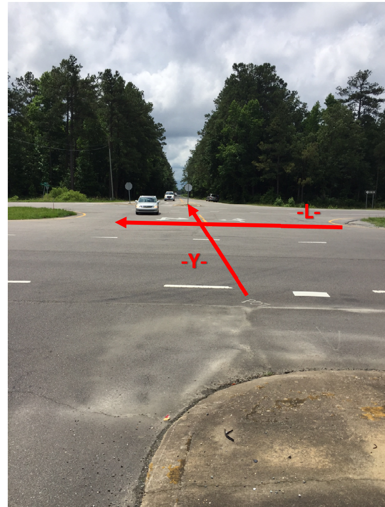
View Looking South from End Bent 1
