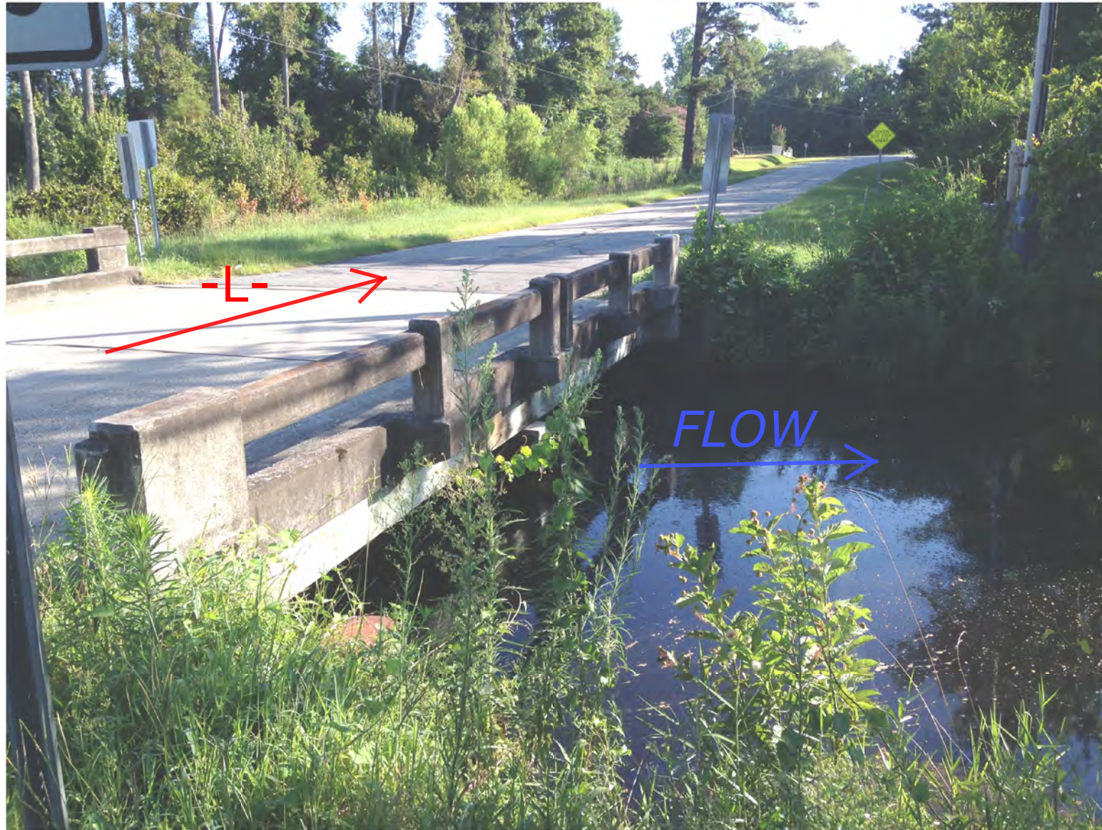
VIEW LOOKING NORTHEAST FROM END BENT 1
