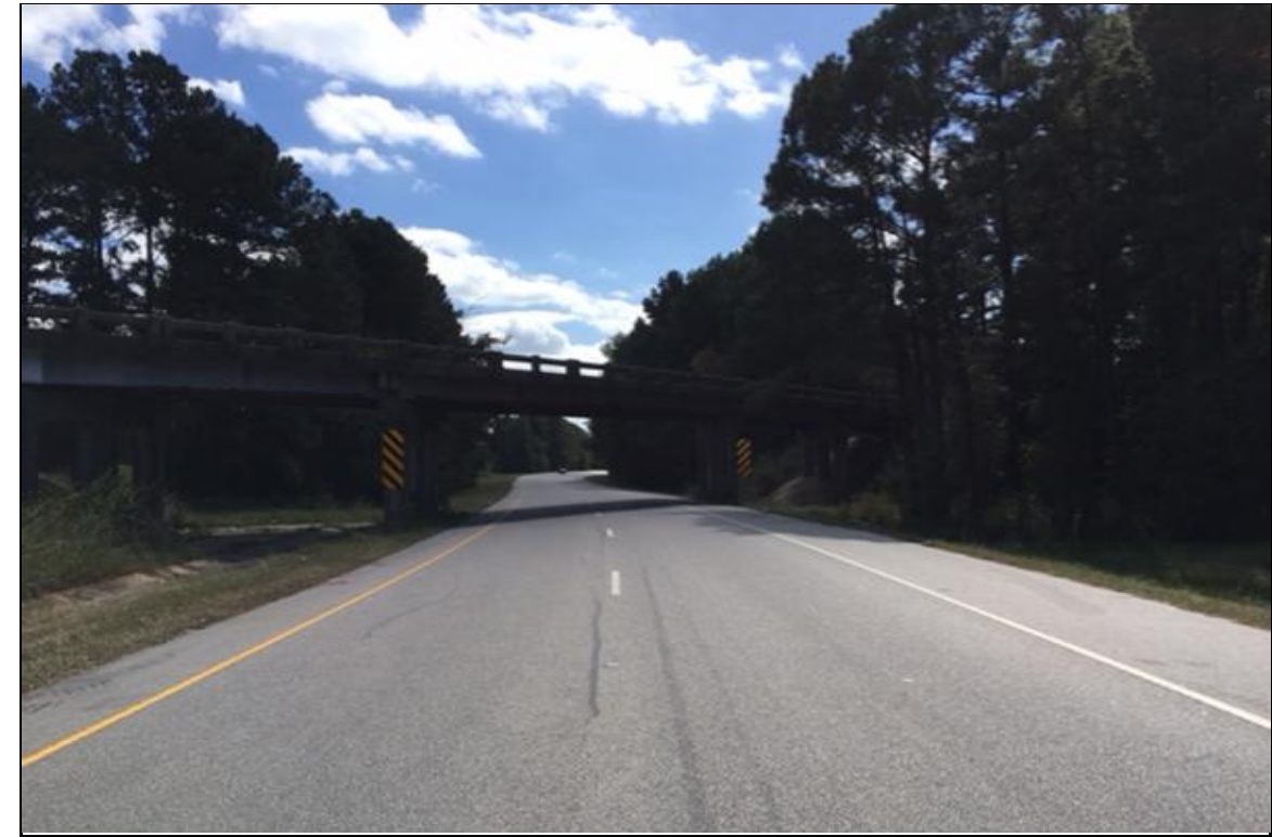
PHOTOGRAPH NO. 3: ON -L2- ALIGNMENT, NORTH OF -L- ALIGNMENT, LOOKING SOUTH
