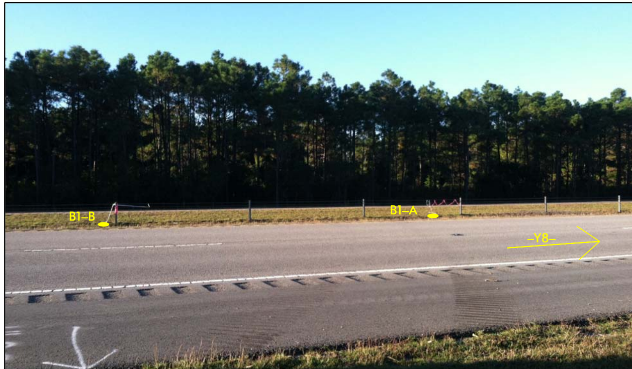
LOOKING DOWNSTATION ALONG -L- TOWARD INTERIOR BENT FROM END BENT 2
