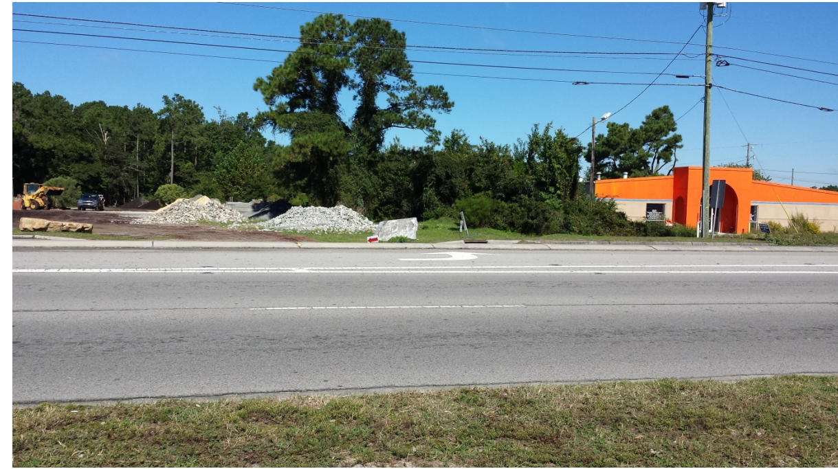
Photograph No. 3: View looking NW across Market Street from End Bent 1 toward End Bent 2
