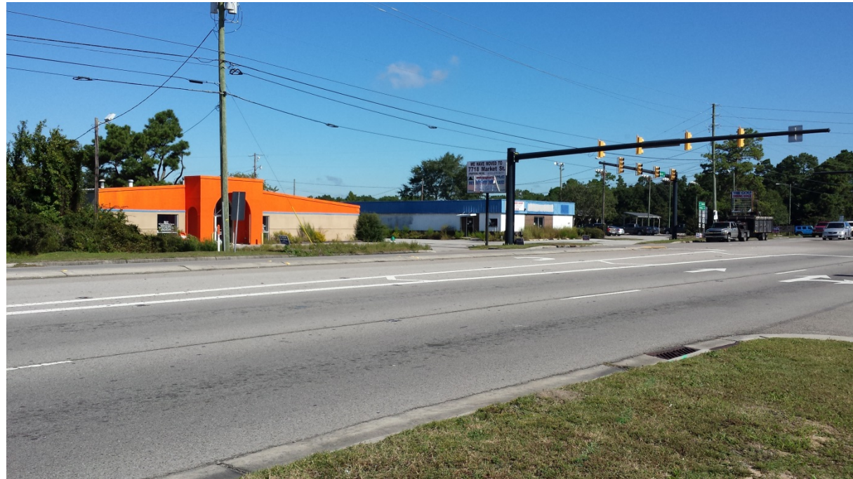
Photograph No. 1: View looking North across Market Street from End Bent 1 toward End Bent 2
