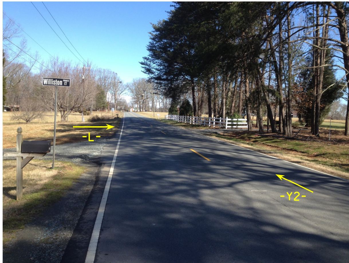
Site Photo No. 1: End Bent 1 -Y2- (Willison Road) Looking Upstation (North)
