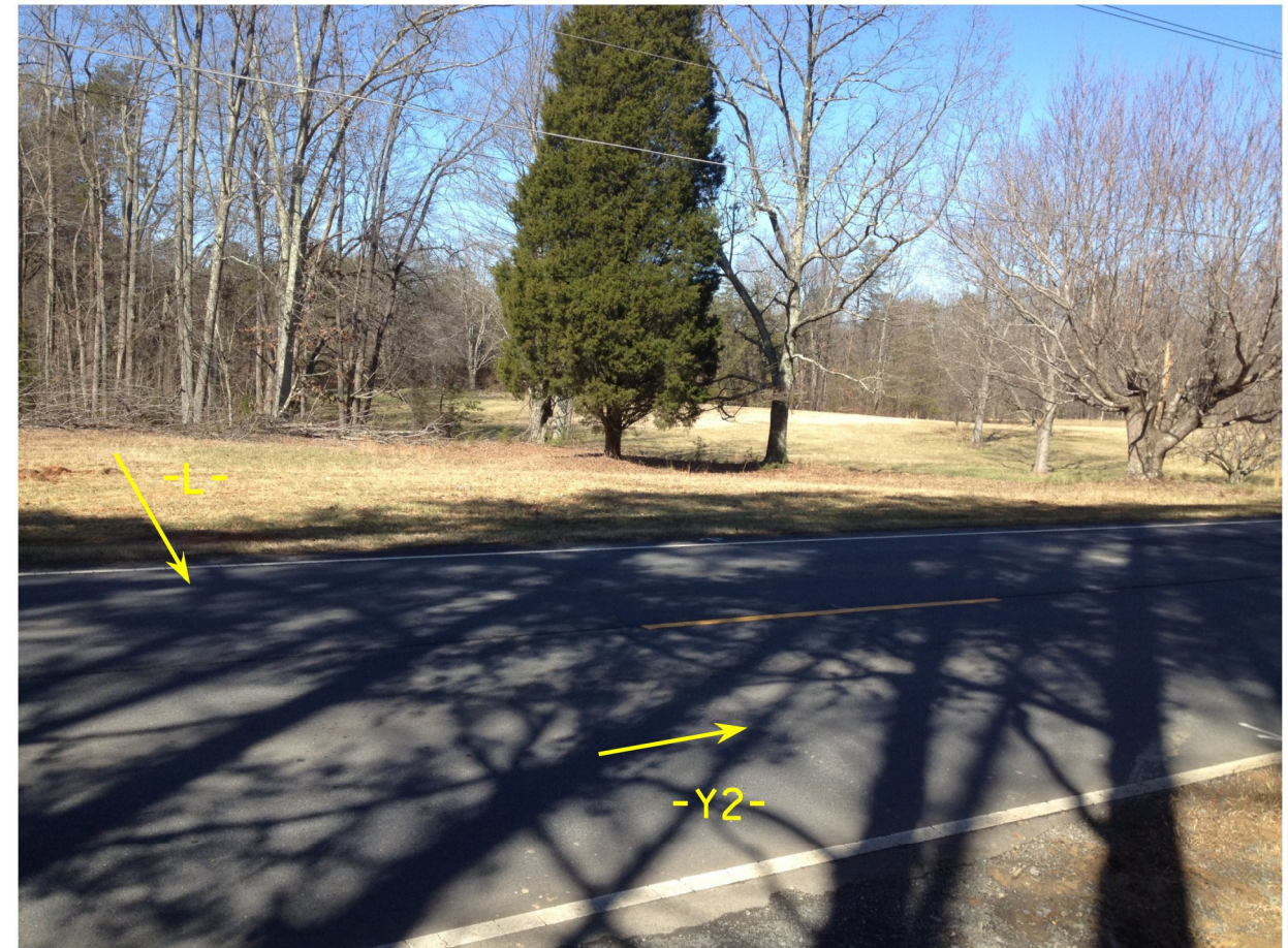
Site Photo No. 3: Bent 1 -L- (Future I-74) Looking Downstation (West)
