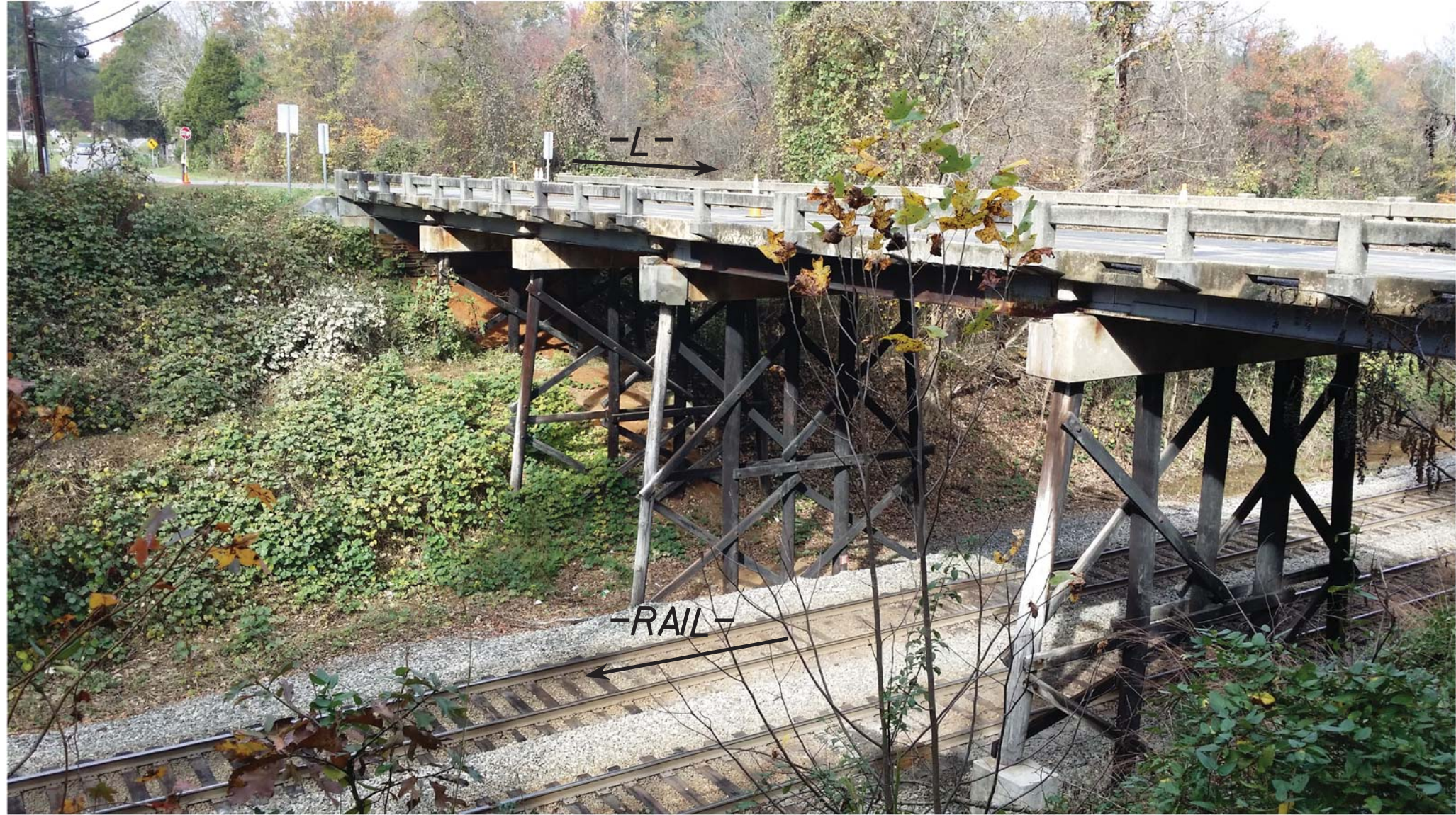
VIEW LOOKING NORTHWEST AT BRIDGE 85
