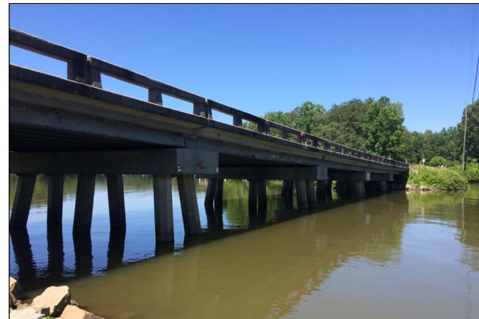
LOOKING DOWNSTATION FROM RIGHT OF EB2, DOWNSTREAM RIGHT.
