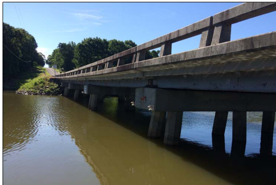
LOOKING UPSTATION FROM LEFT OF EB1, DOWNSTREAM LEFT.
