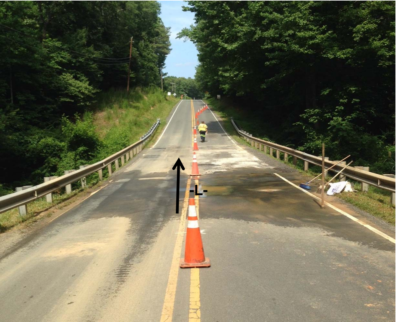
View of SR 1005 looking east
