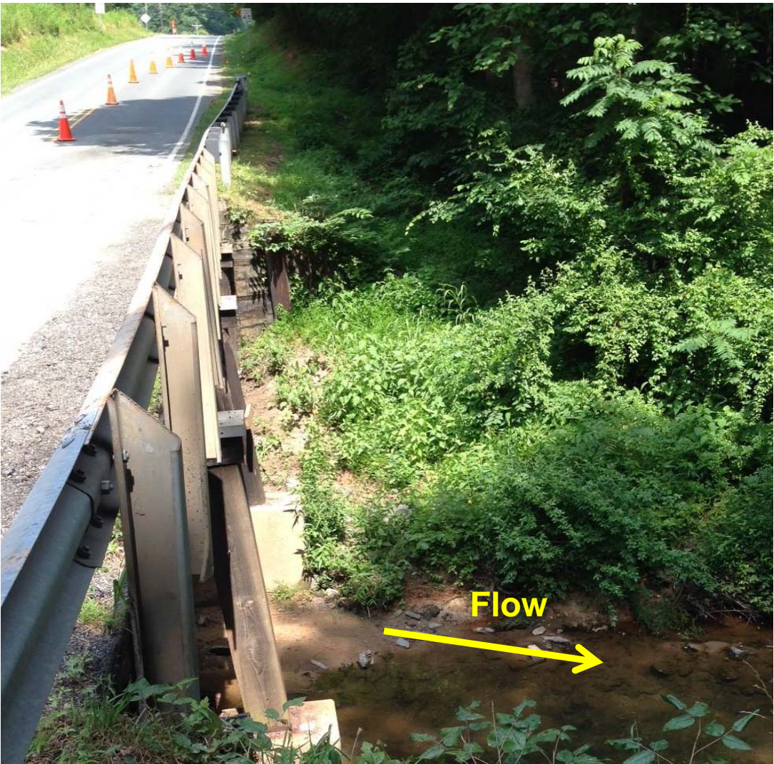
View of Bridge No. 85 looking east
