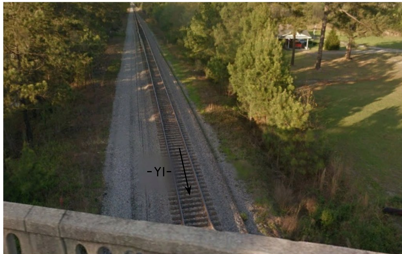
Site Photo No. 2: -YI- (CSX RR) Looking Downstation (East)
