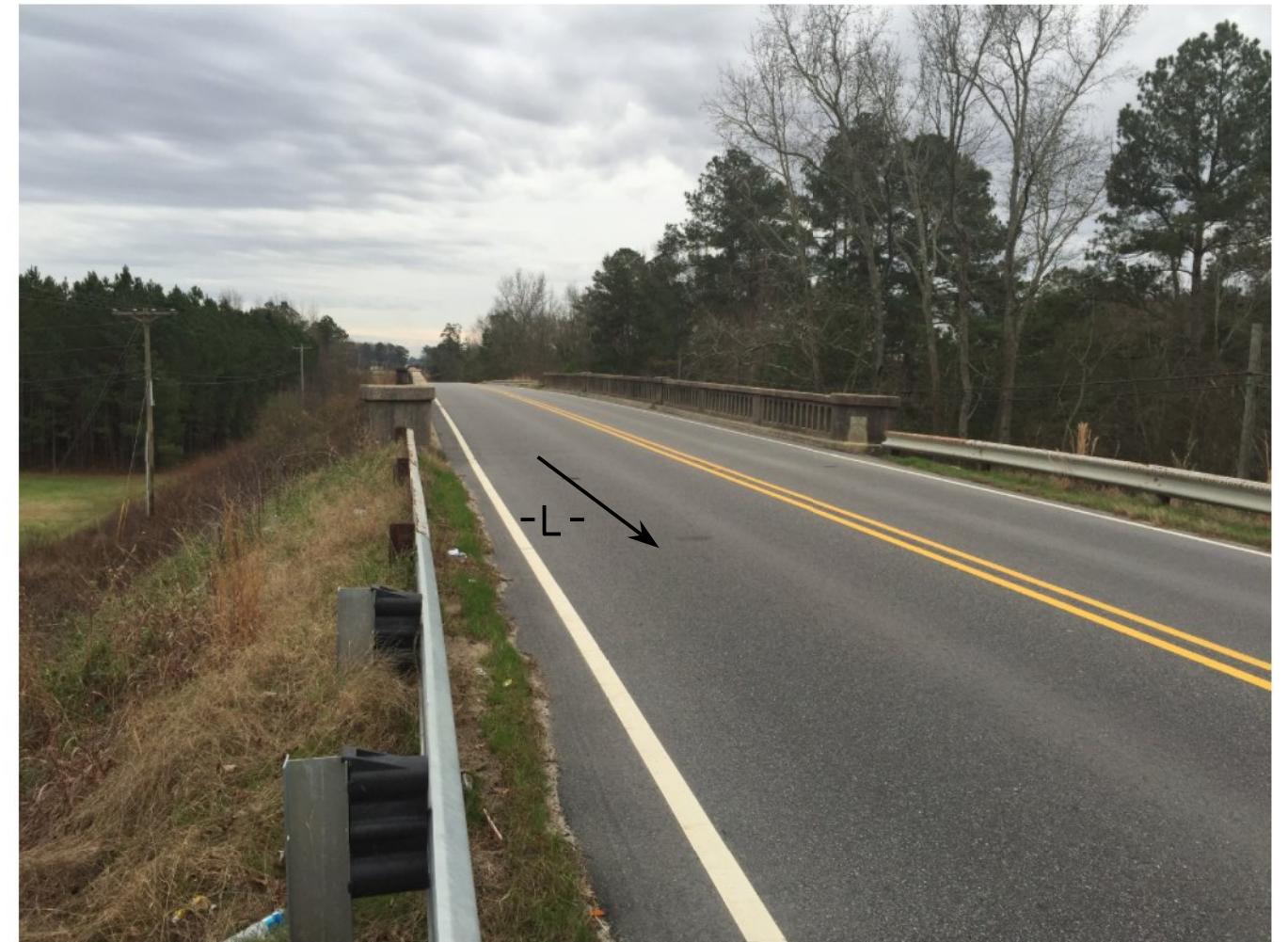
Site Photo No. 3: -L- (NC 211) Looking Downstation (North)
