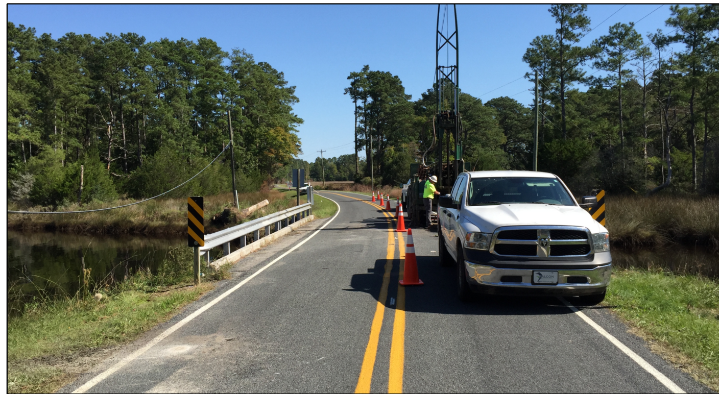
LOOKING UPSTATION ALONG -L-. DRILL RIG SETUP ON B1-B. EB1-A COMPLETED AND VISIBLE FOREGROUND LEFT.
