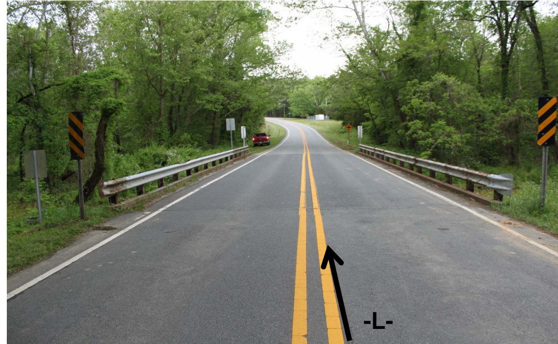
View of SR 2136 looking northwest.
