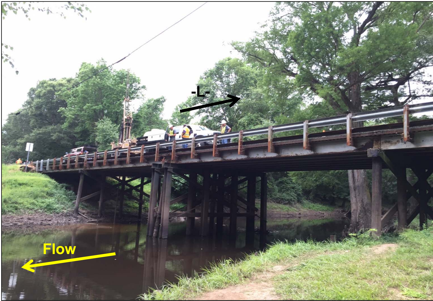
View of Bridge No. 11 looking southwest
