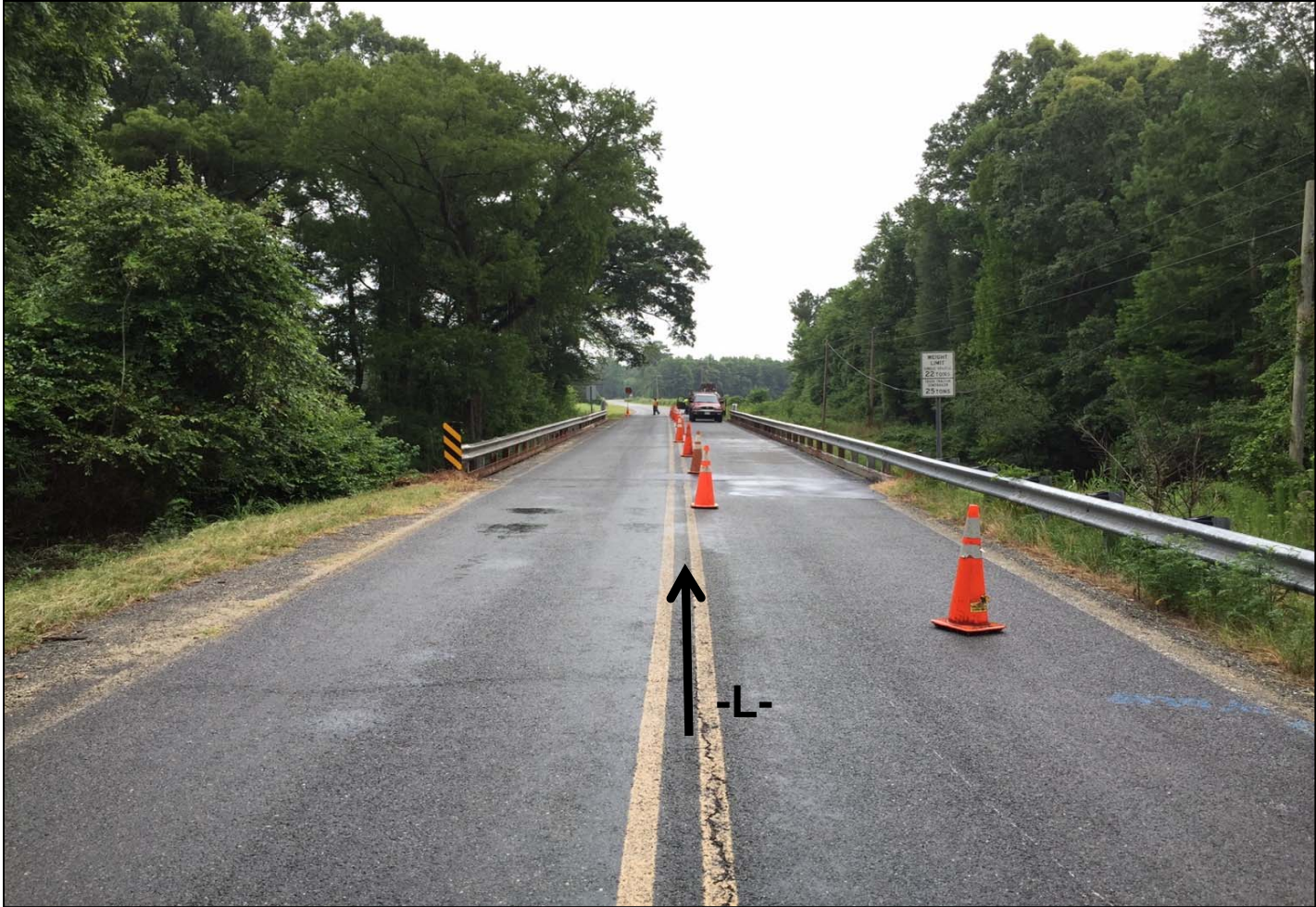
View of SR 1201 looking northeast
