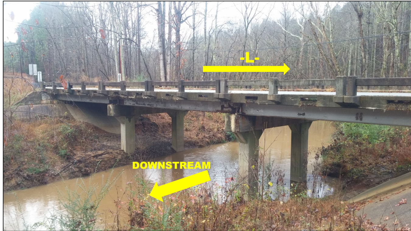
GRASSY CREEK, LOOKING UPSTREAM TOWARDS EXISTING BRIDGE.
