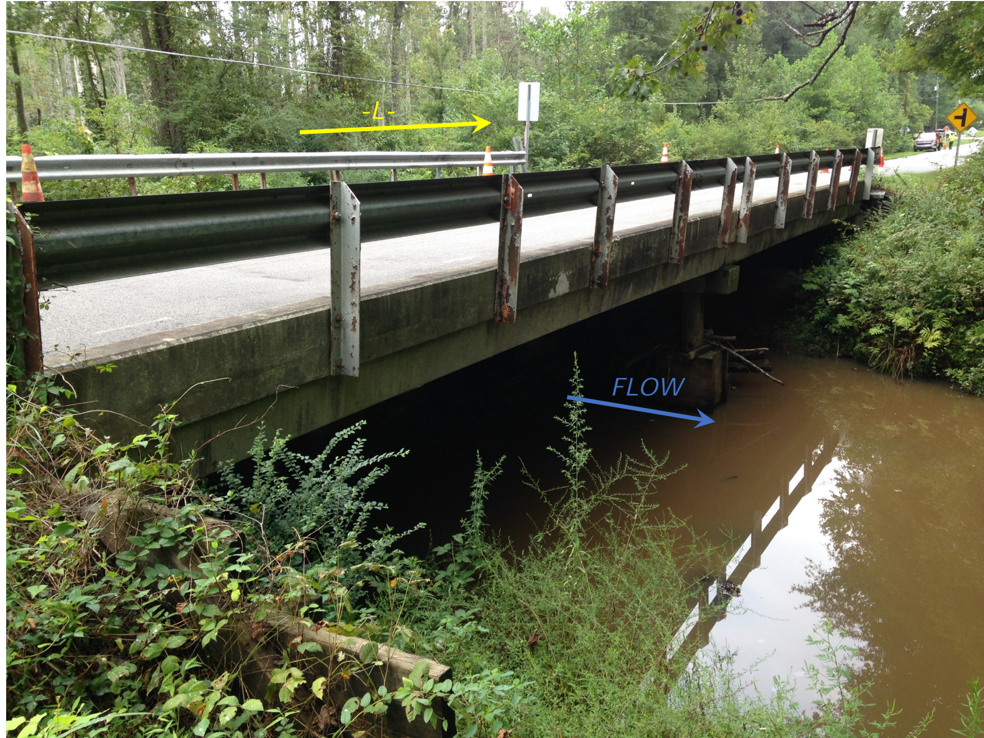
VIEW ALONG EAST SIDE OF BRIDGE LOOKING NORTH
