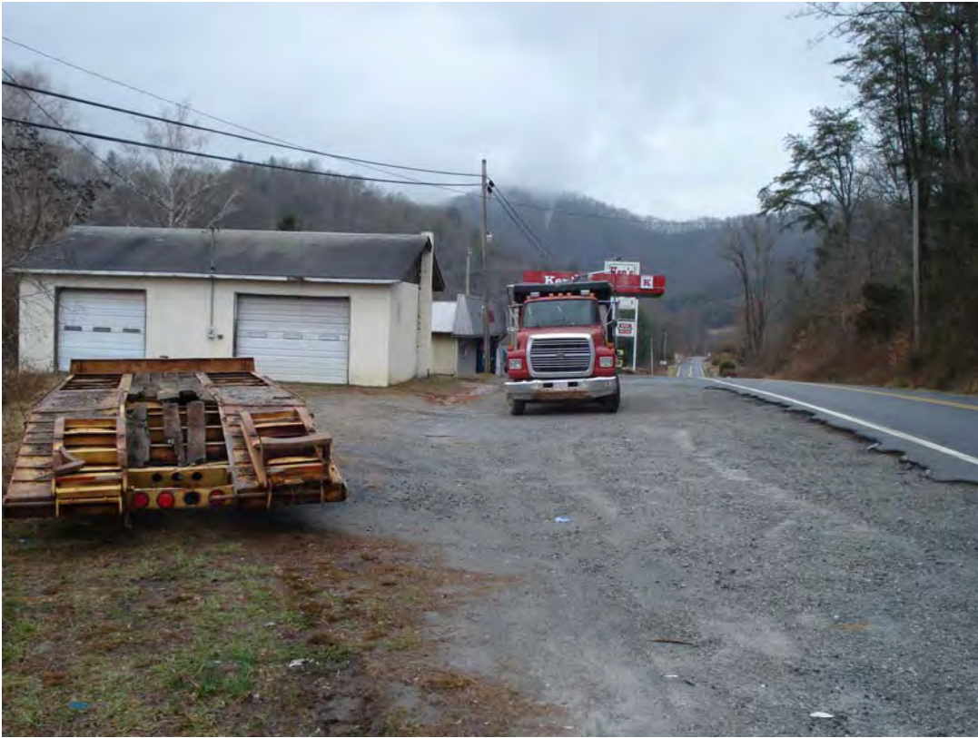
Photograph 1 : View looking north at suspected former auto repair facility located on Parcel 071.
