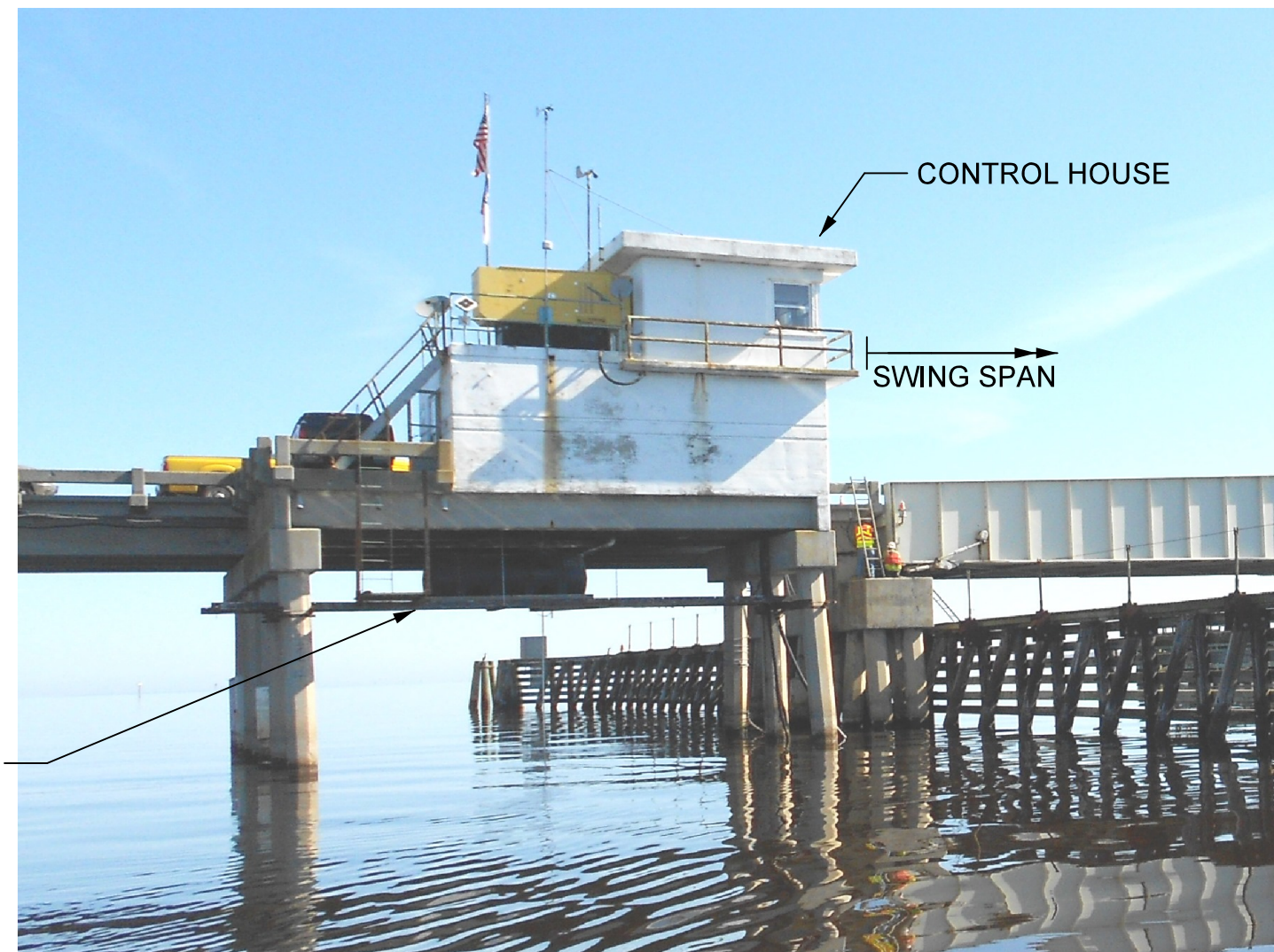
SEPTIC TANK PLATFORM
