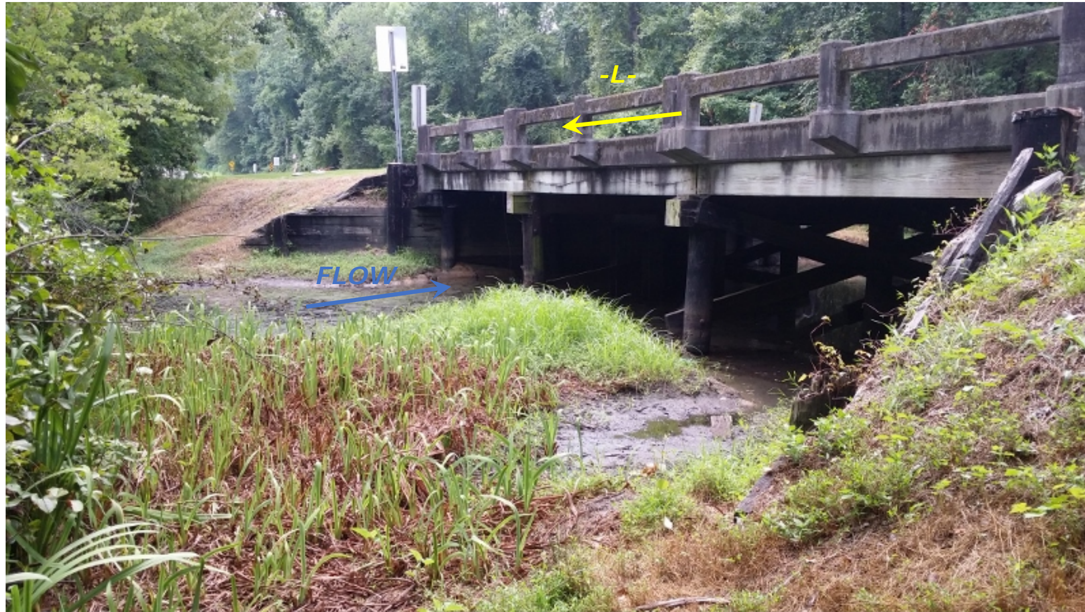
VIEW ALONG NORTH SIDE OF BRIDGE LOOKING SOUTHEAST
