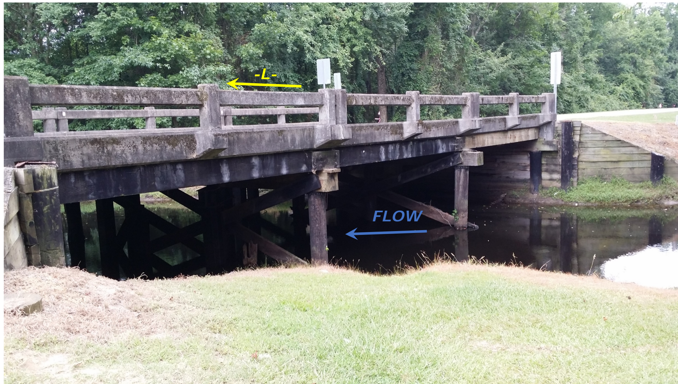
VIEW ALONG NORTH SIDE OF BRIDGE LOOKING SOUTHWEST
