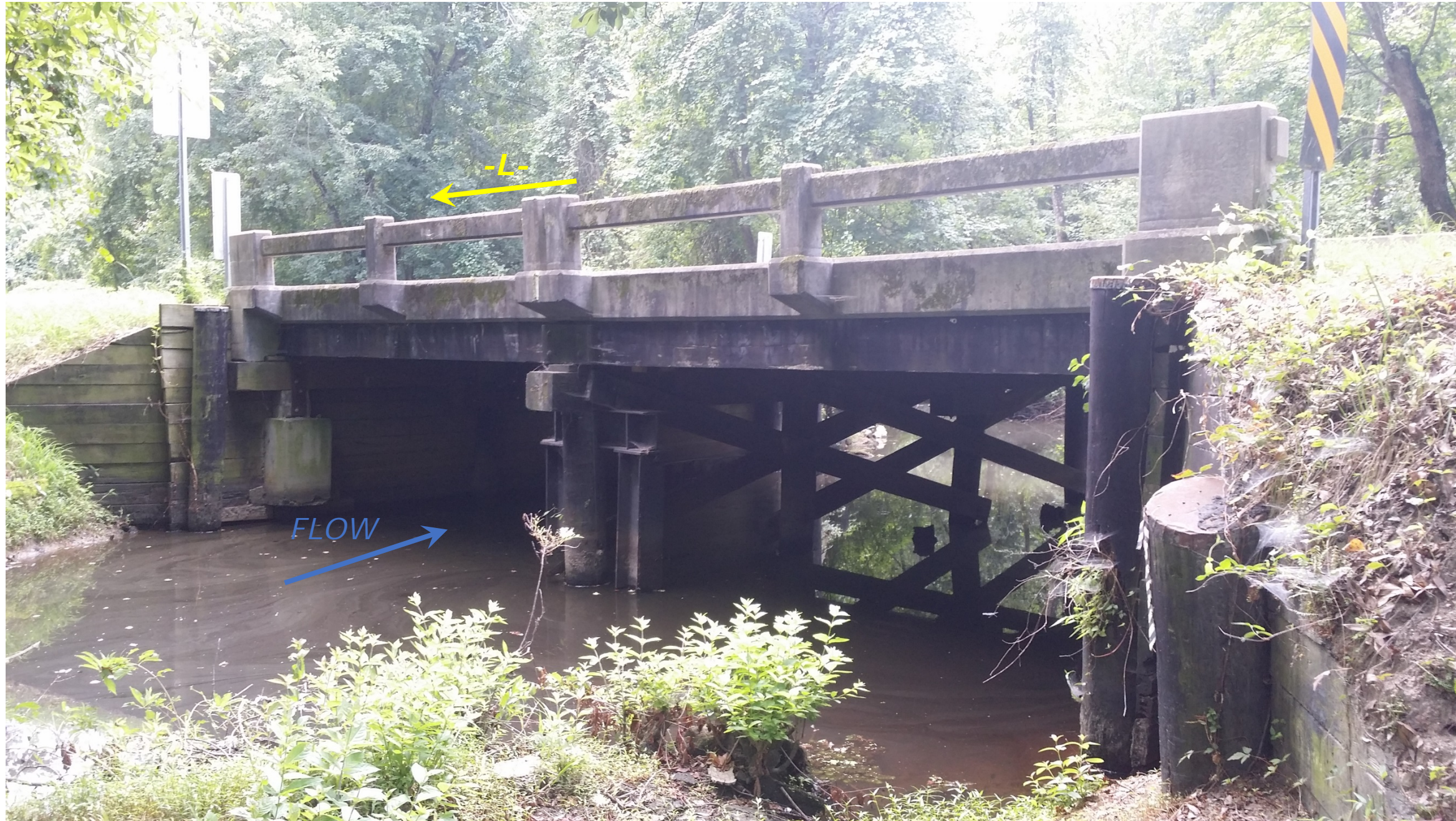
VIEW ALONG EAST SIDE OF BRIDGE LOOKING NORTH
