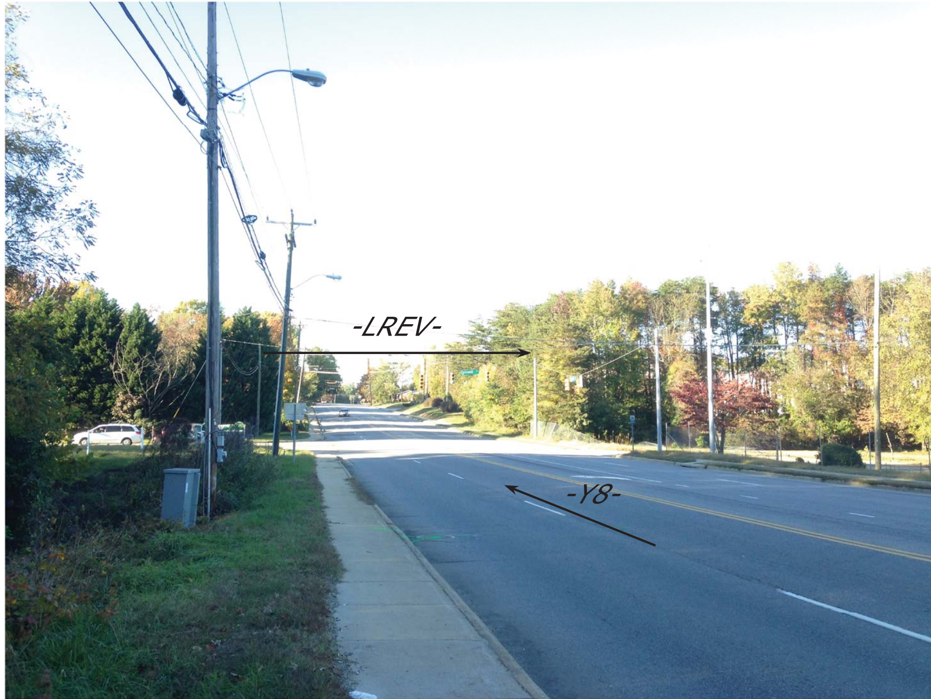
VIEW ALONG -Y8- (LAWNDALE DR.) LOOKING NORTH
