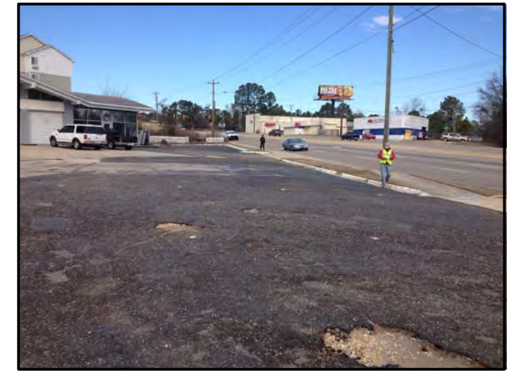
View of Northeast Portion of Survey Area (Facing Approximately North)
