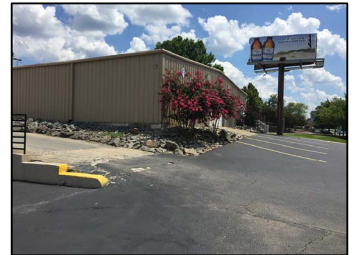
View of South Survey Area (Facing Approximately South)
