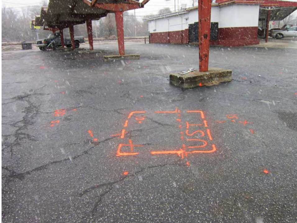
Parcel 020 (Unassigned AKA P&S Enterprises Property), looking east. Photo shows approximate marked location of Probable UST No. 1 near the southwest end of the canopy on Parcel 020.
