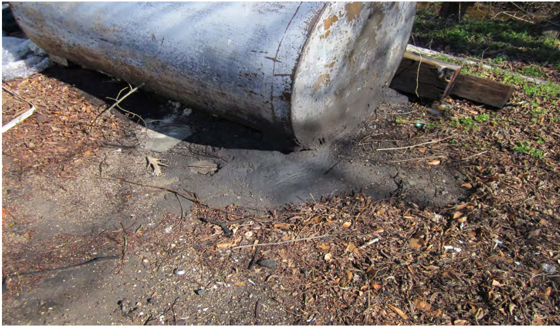
Parcel 007, facing east. Above-ground storage tank with staining at base and "Used Oil" sticker on tank.
