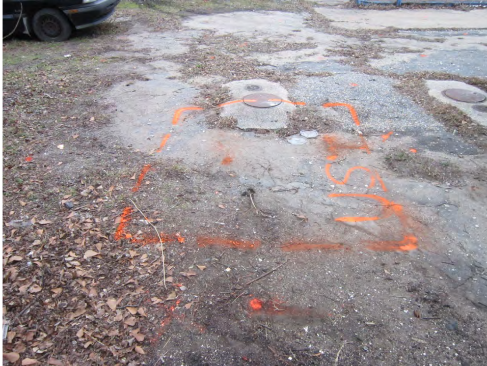
Parcel 007 (Edmund George Property), looking south. Photo shows approximate marked location of Probable UST No. 3 near the southeast corner of the building on Parcel 007.
