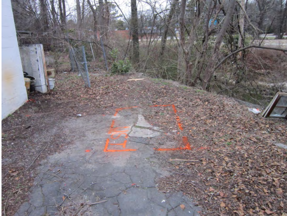
Parcel 007 (Edmund George Property), looking north. Photo shows approximate marked location of Probable UST No. 1 near the northeast corner of the building on Parcel 007.
