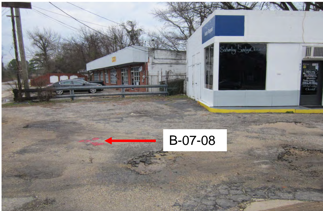
Parcel 007, facing north toward B-07-08.
