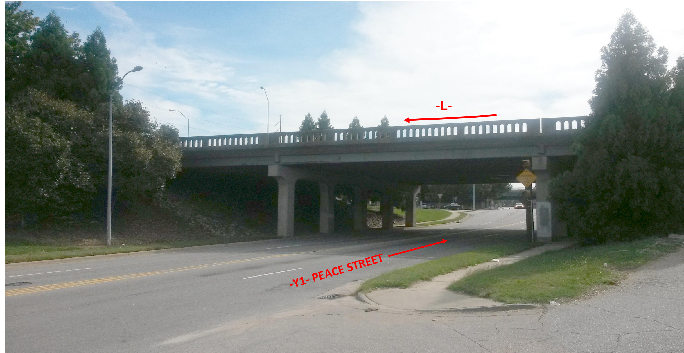
LOOKING EAST TOWARD END BENT 2
