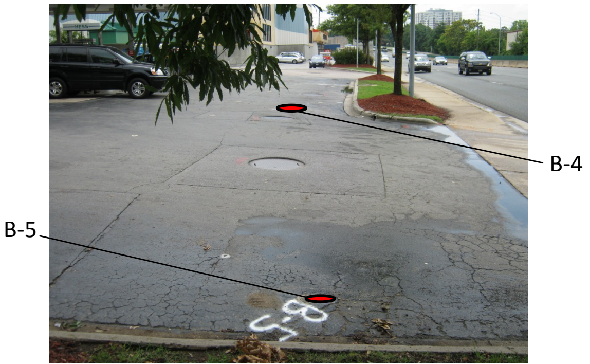
Photo #3: Boring locations B-4 and B-5, facing south.
