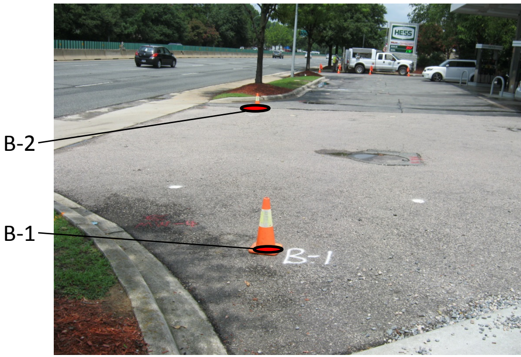
Photo #1: A view of Borings B-1 and B-2, facing north.
