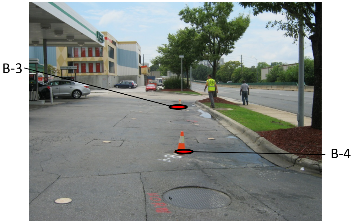
Photo #2: A view of Borings B-3 and B-4, facing south
