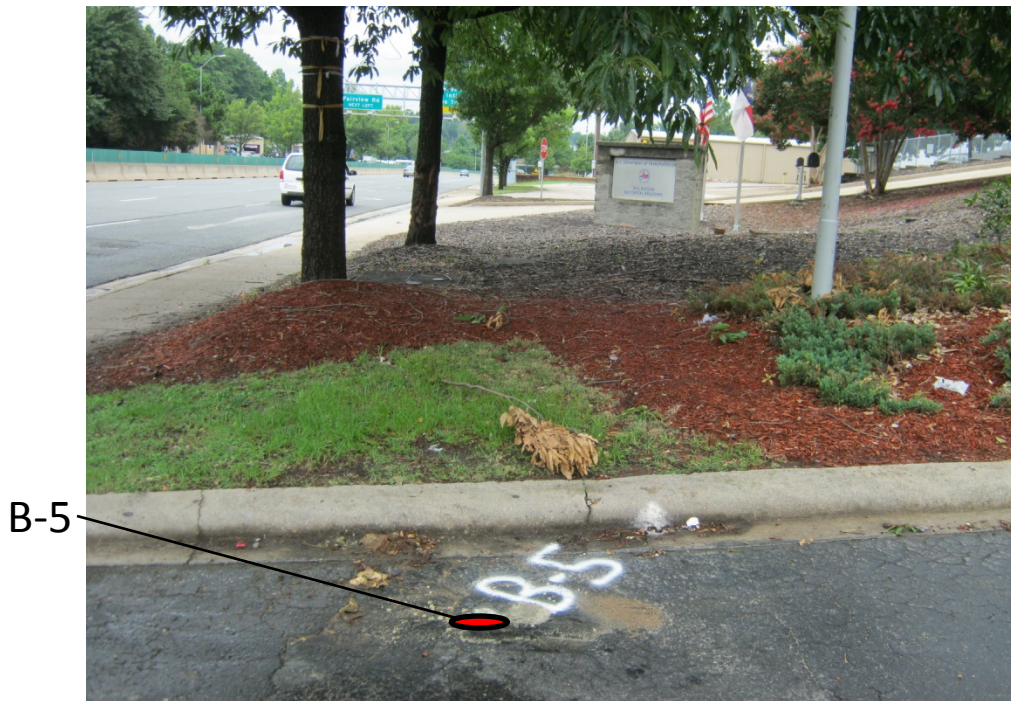
Photo #4: A view of boring location B-5, facing north.
