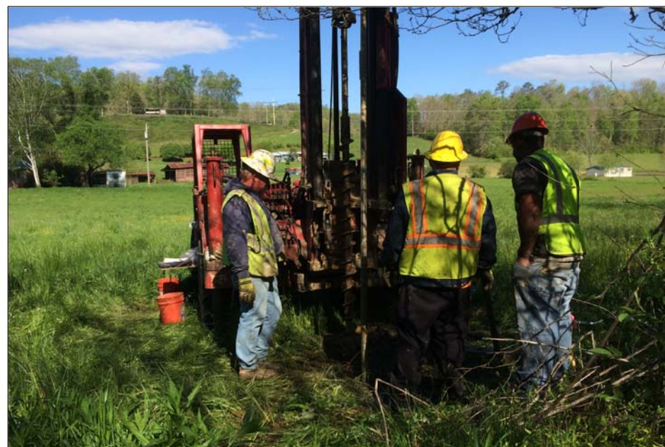
DRILL RIG SET UP ON EB1-A
