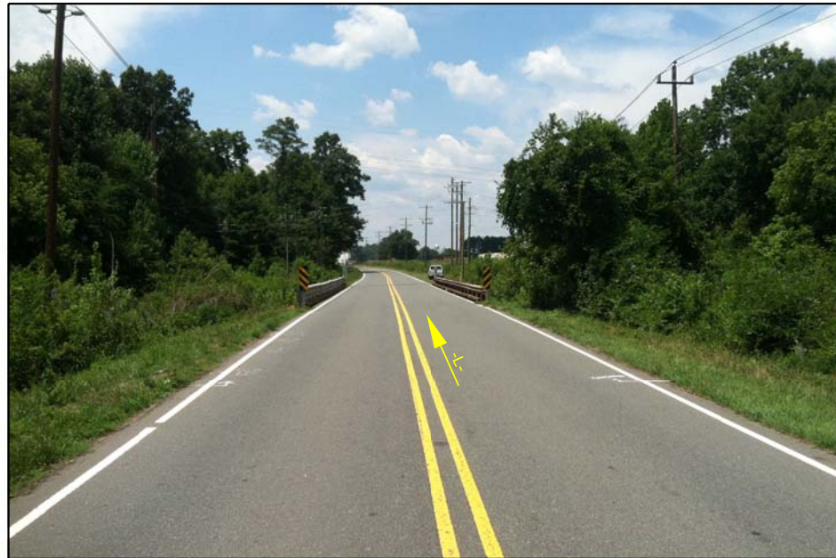
PHOTOGRAPH TAKEN ON SR 1916 (CORINTH RD) LOOKING UPSTATION ALONG ALIGNMENT -L-
