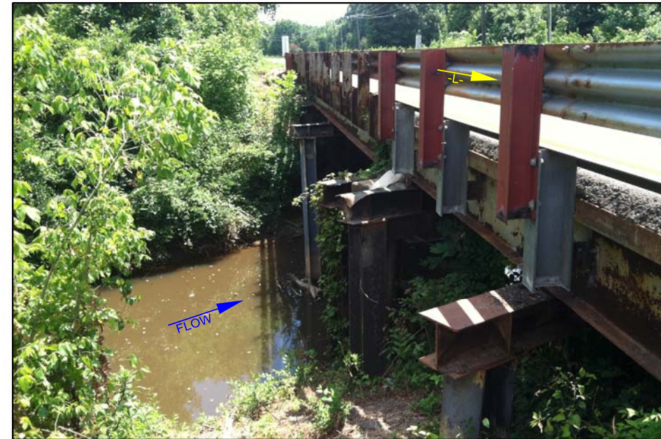
PHOTOGRAPH TAKEN FROM END BENT 2 LOOKING DOWNSTATION ALONG -L-
