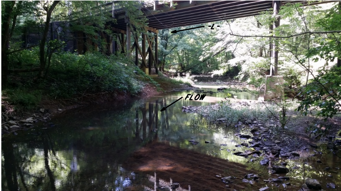
PHOTOGRAPH 1: VIEW OF AARON'S CREEK BELOW BRIDGE I25 LOOKING UPSTREAM.
