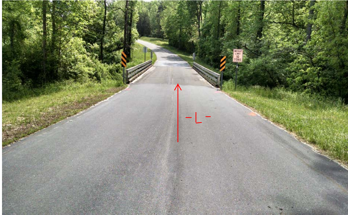
View of Existing Bridge No. 178 Looking Upstation
