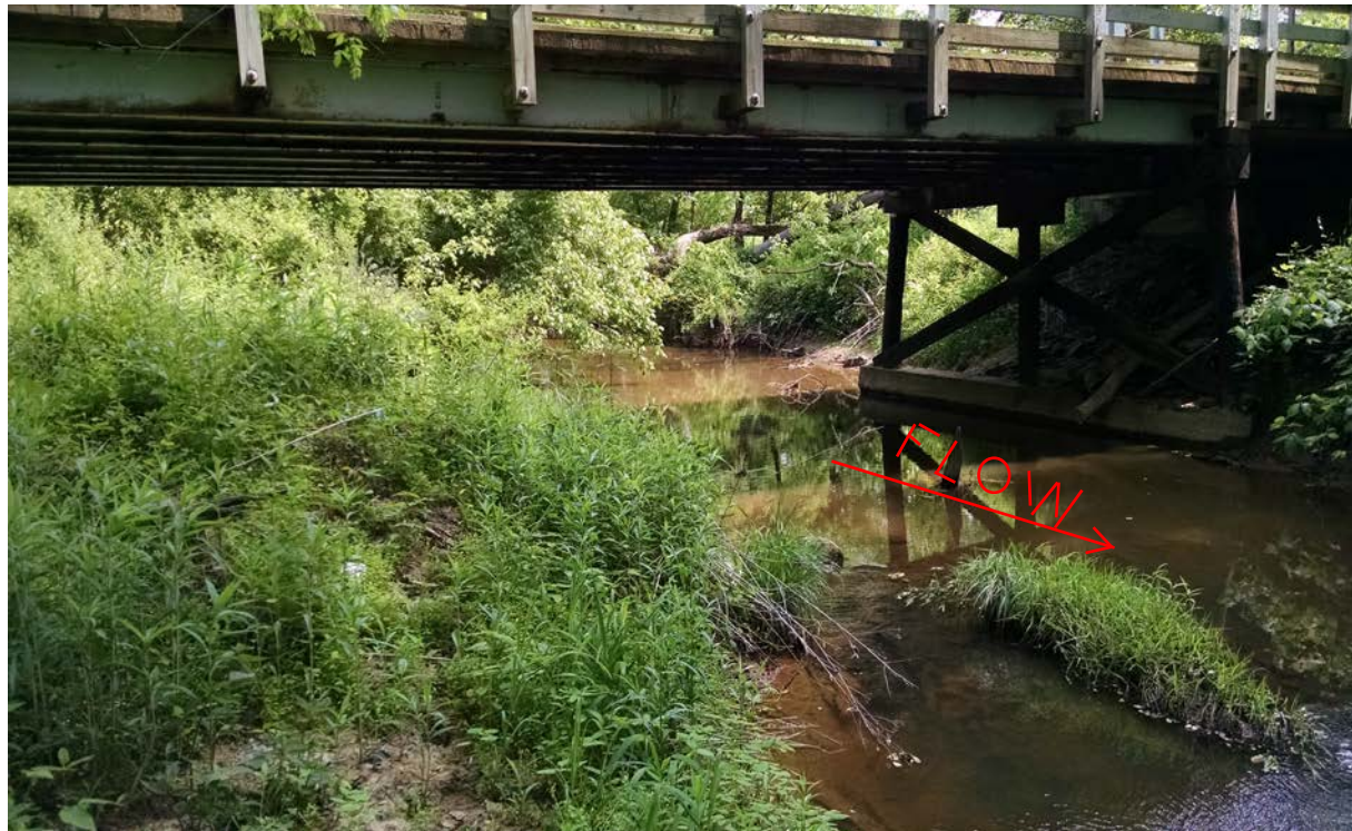
View of Existing Bridge No. 178 Looking Upstream
