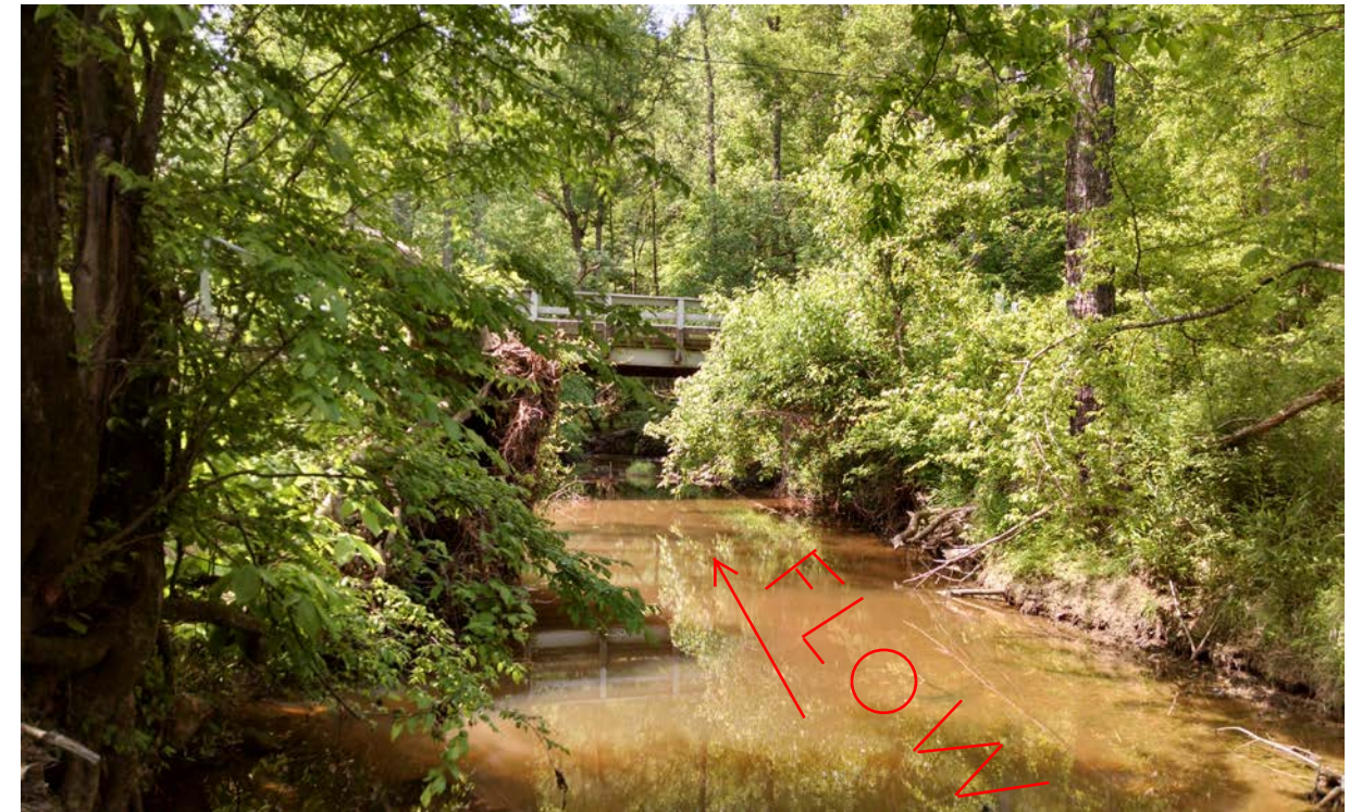
View of Existing Bridge No. 178 Looking Downstream
