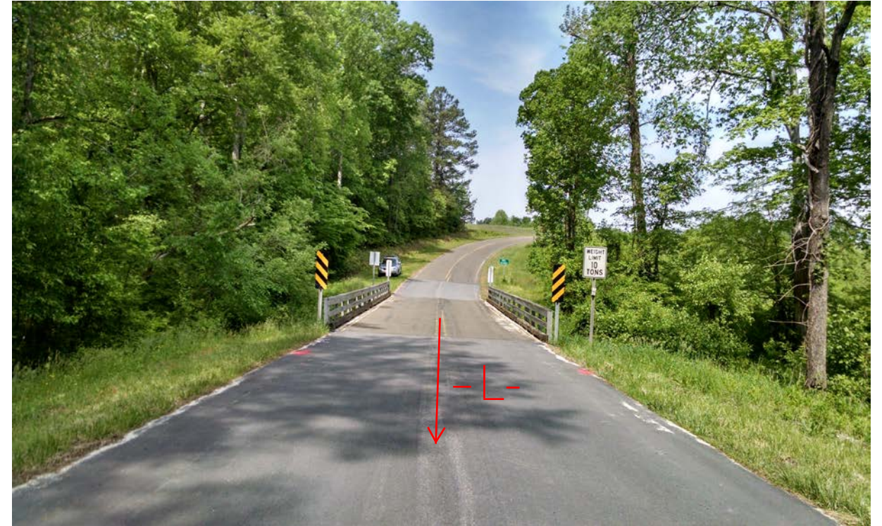
View of Existing Bridge No. 178 Looking Downstation
