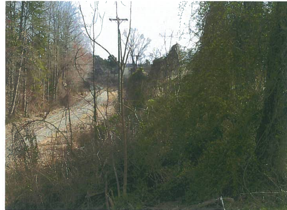
Photograph No.2: This photograph was taken from the right side of the -Y- alignment looking East across proposed Interior Bent No. 2.
