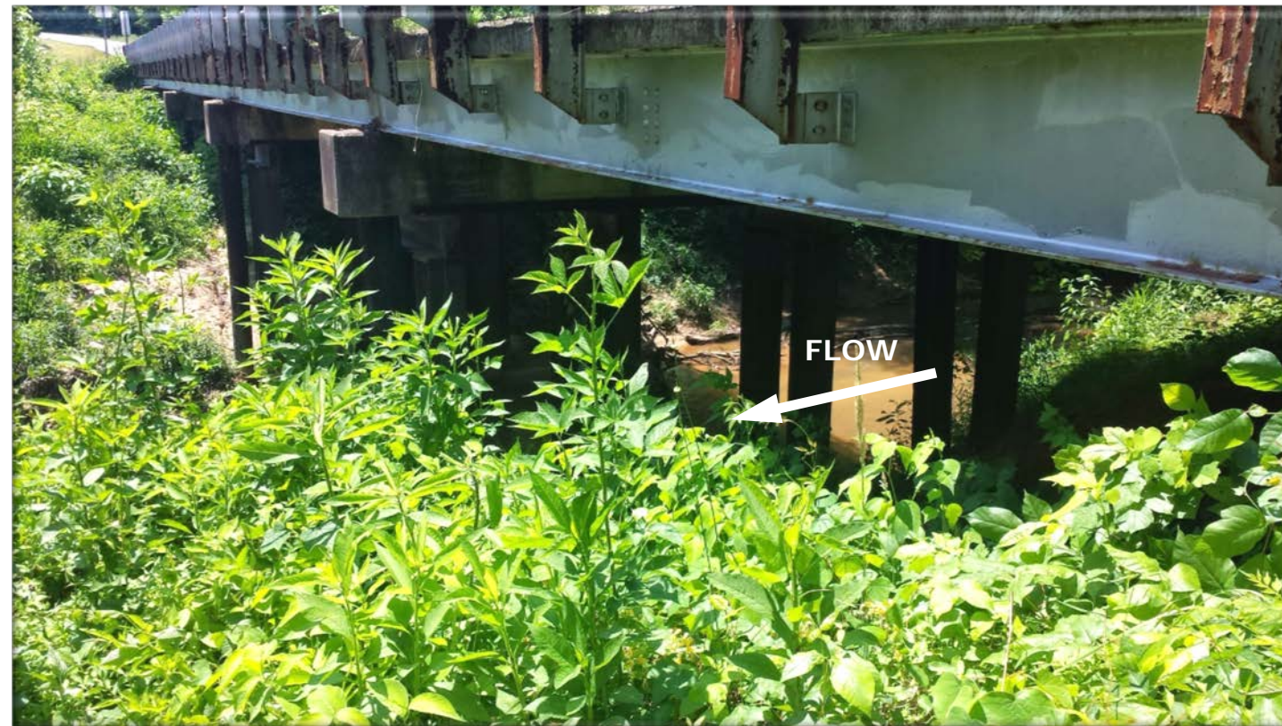
PHOTOGRAPH 2: VIEW OF EAST SIDE OF BRIDGE 110 FROM NORTH END.
