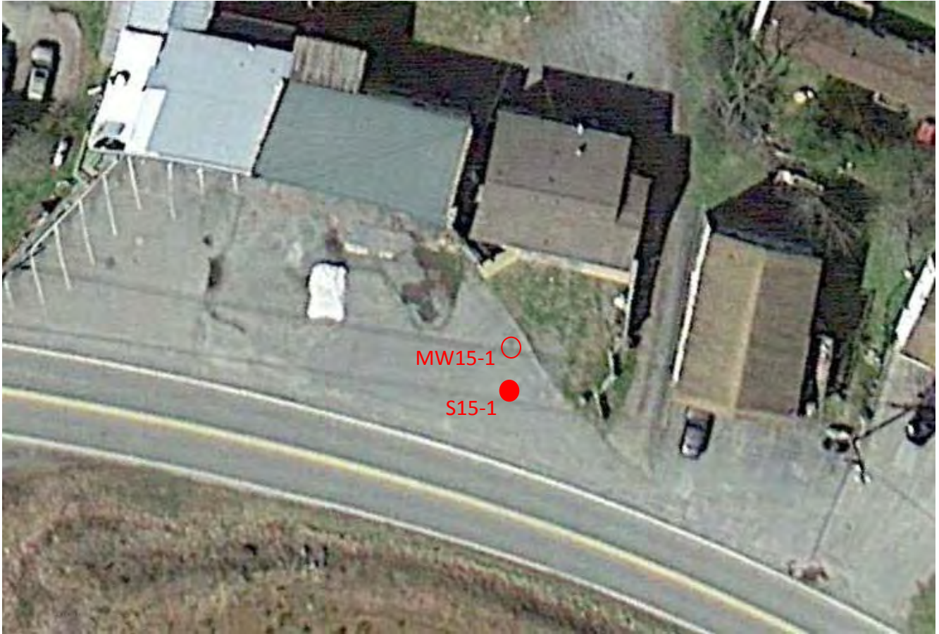
Photograph 1: Aerial view showing boring location S15-1 and existing monitoring well MW15-1 on Parcel 015. West is at the top of photo (aerial is from Google Earth).
