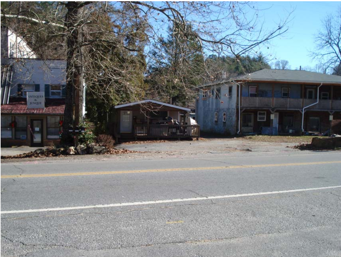
Photograph 3 : View looking southeast at detached 1-story office building.
