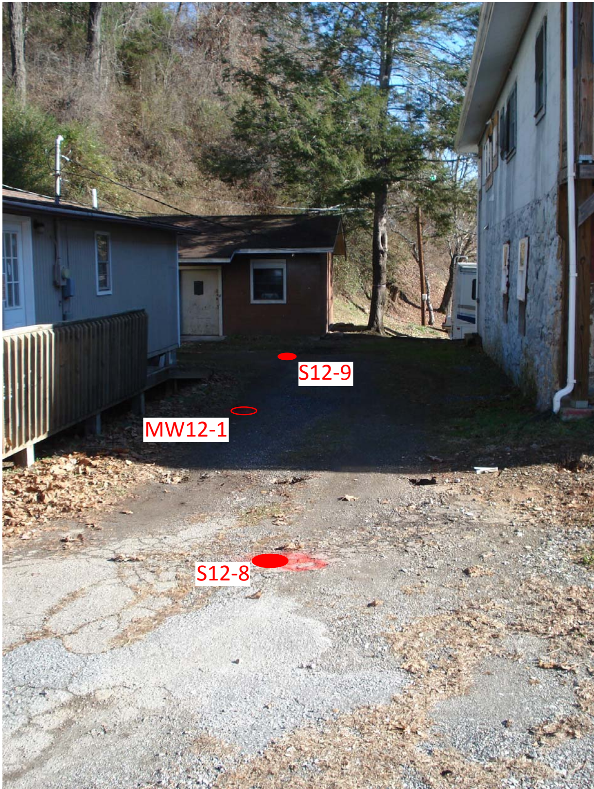
Photograph 6 : View looking southwest at soil boring locations S12-8 and S12-9, and existing groundwater monitoring well location MW12-1. Detached storage building is shown in the background.
