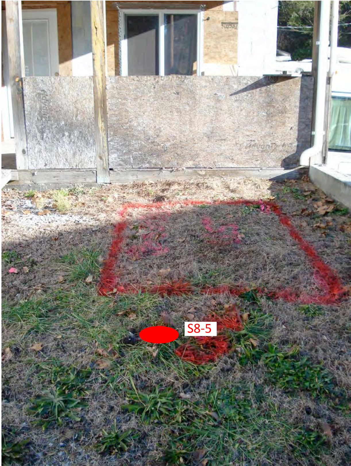
Photograph 5: View looking north at "Probable UST" and boring location S8-5 at Parcel 008.
