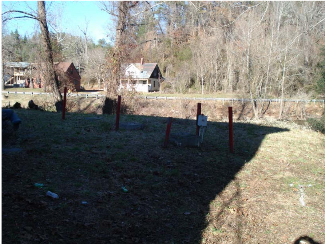
Photograph 5 : View looking north at septic tanks and sewage pump station located west of soil boring S6-6. The Tuckasegee River and Edgewater Road are shown in the background.
