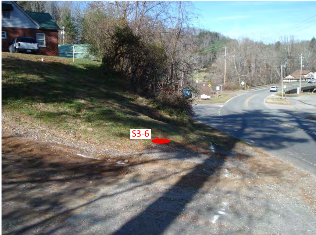
Photograph 5: View looking north at soil boring location S3-6 at Parcel 003. Old Cullowhee Road is shown on right, and bridge over Tuckasegee River is shown in the background.
